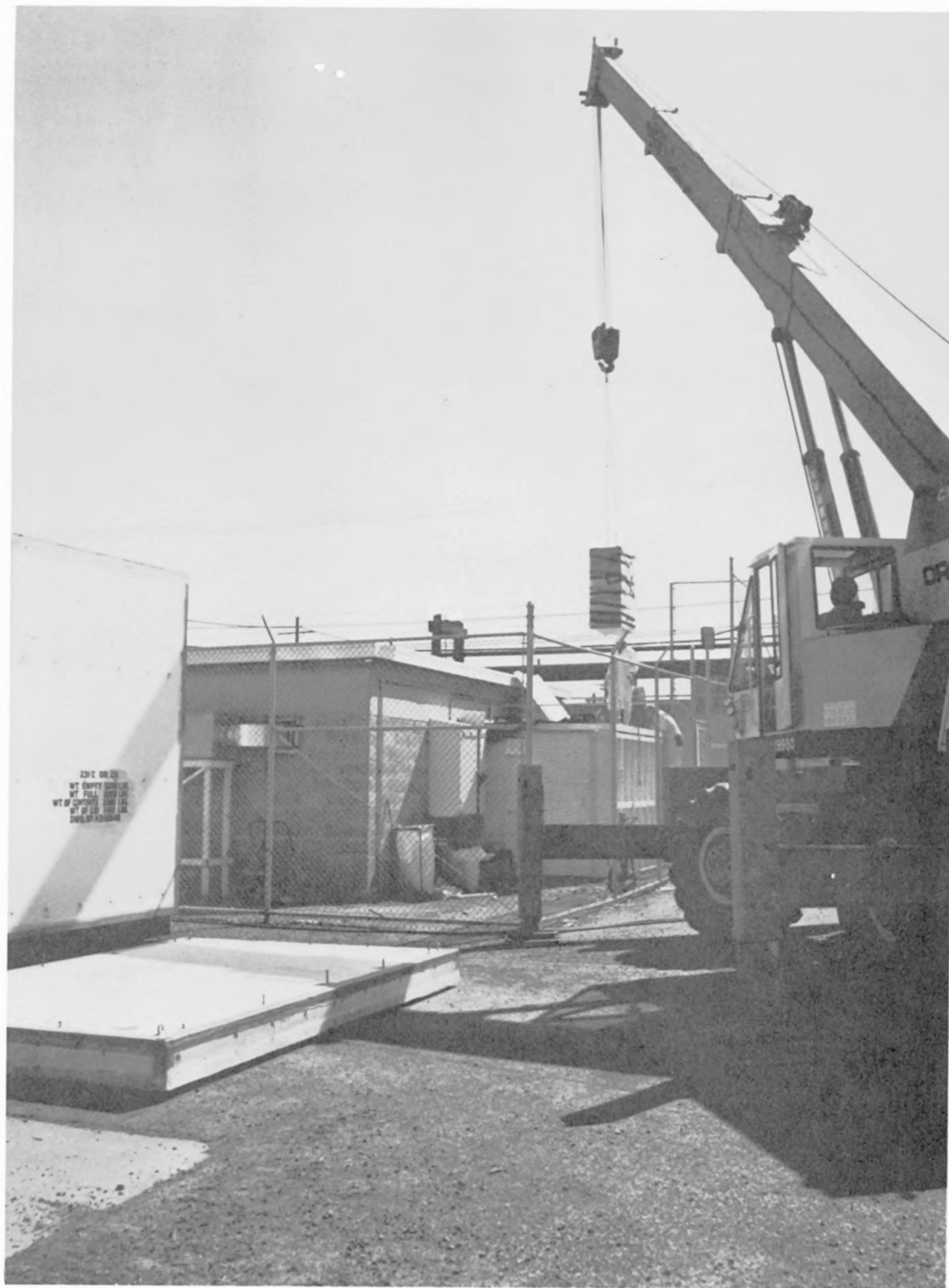
FIGURE 10. Removal of Packaged Contaminated Objects from 303-C Building T-18
