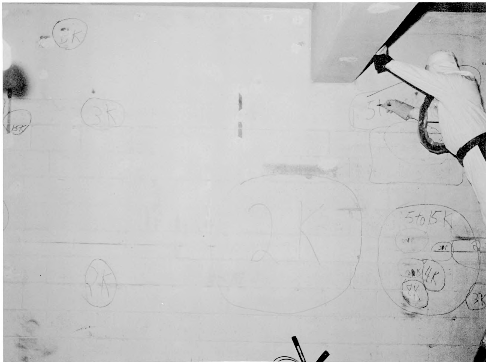
FIGURE 15. Areas of Block Wall in 303-C Building That Could Not be Decontaminated
