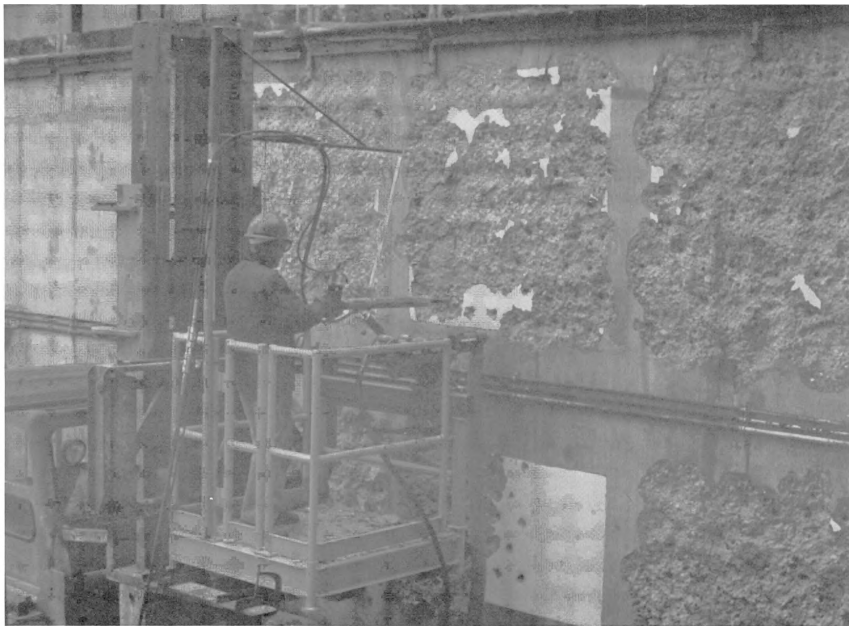
FIGURE 19. Example of the Concrete Spalling Technique Used in 303-C Building Decontamination
