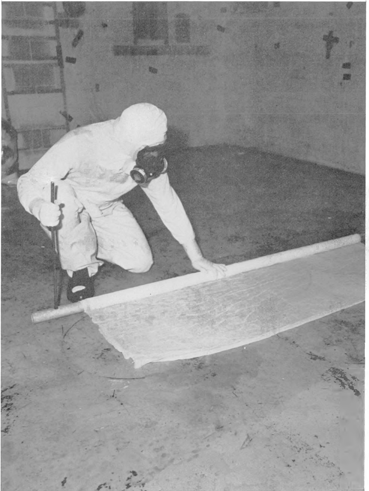
FIGURE 13. Preparation of Cheese Cloth-Strip Coat Decontamination Technique Assembly
