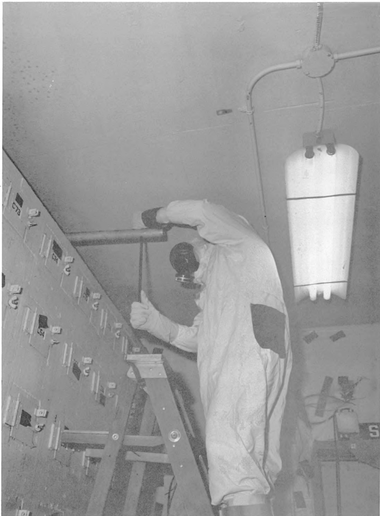
FIGURE 14. Application of Cheese Cloth-Strip Coat Decontamination Technique in the 303-C Building
