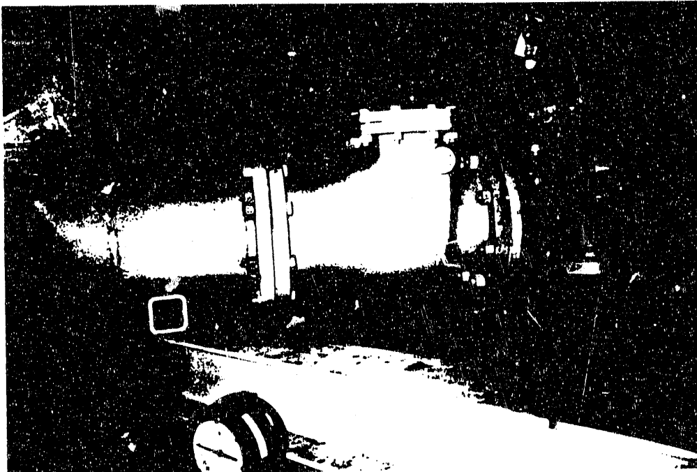
Figure 12. Typical diesel generator check valve installation.
