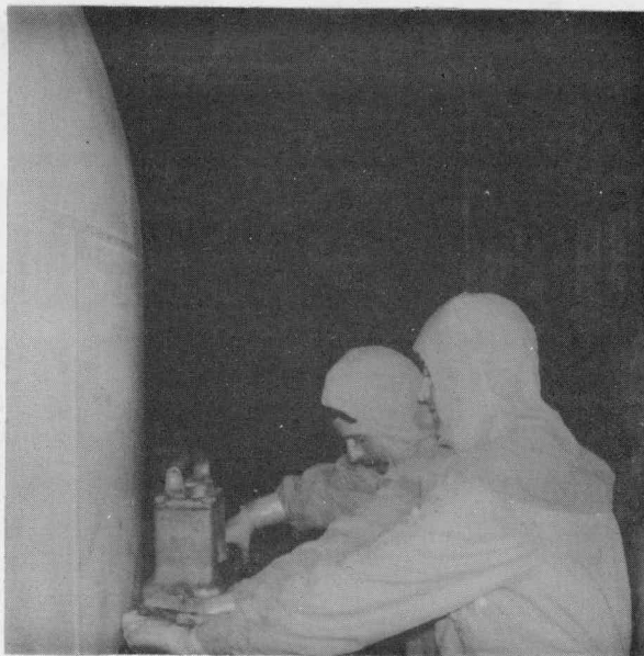
Figure 36. Lowering Drywell Head Bolt Removal Tools into Reactor Cavity (Browns Ferry)
