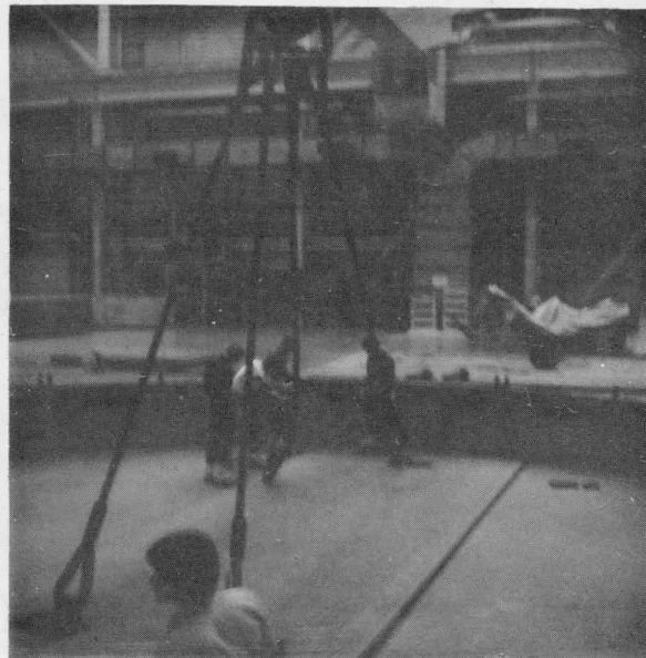
Figure 32. Center - Stuck on Far Corner Using Pry Bar to Loosen (Hatch)
