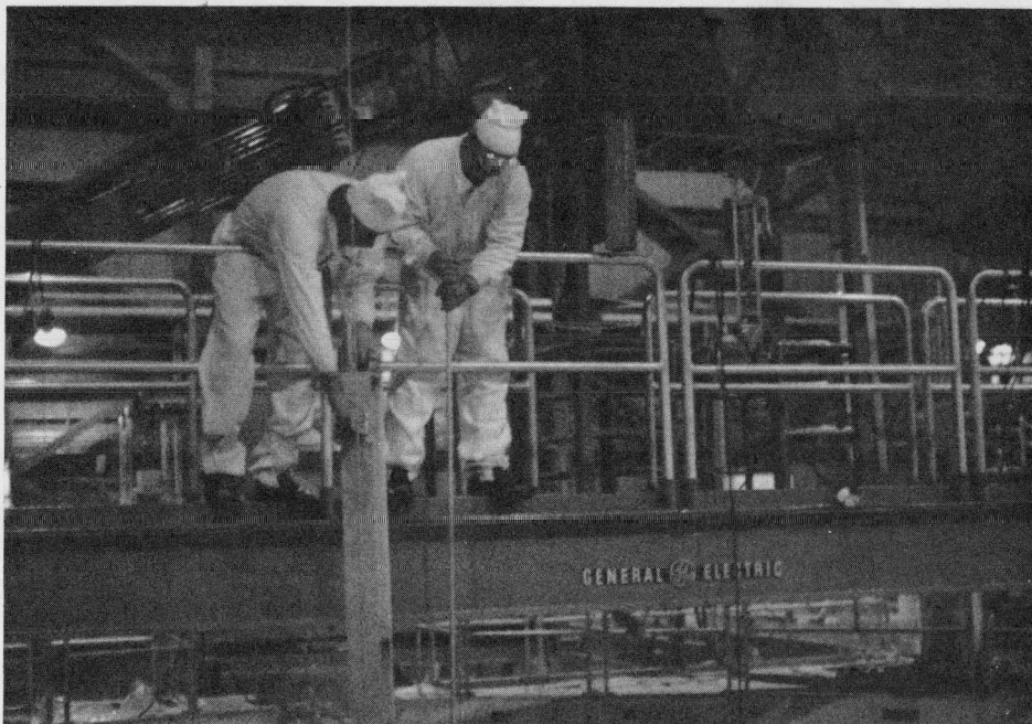
Figure 166. New LPRM has been Removed from Strongback - Will now be Placed in LPRM Holding Tool (Fitzpatrick)
