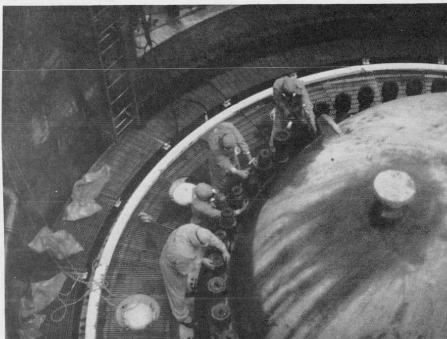
Figure 63. Spinning Off Head Nuts by Hand (Browns Ferry)
