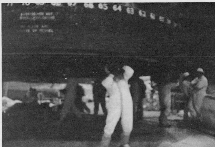
Figure 68. Removing Head Flange O-Ring (Browns Ferry)
