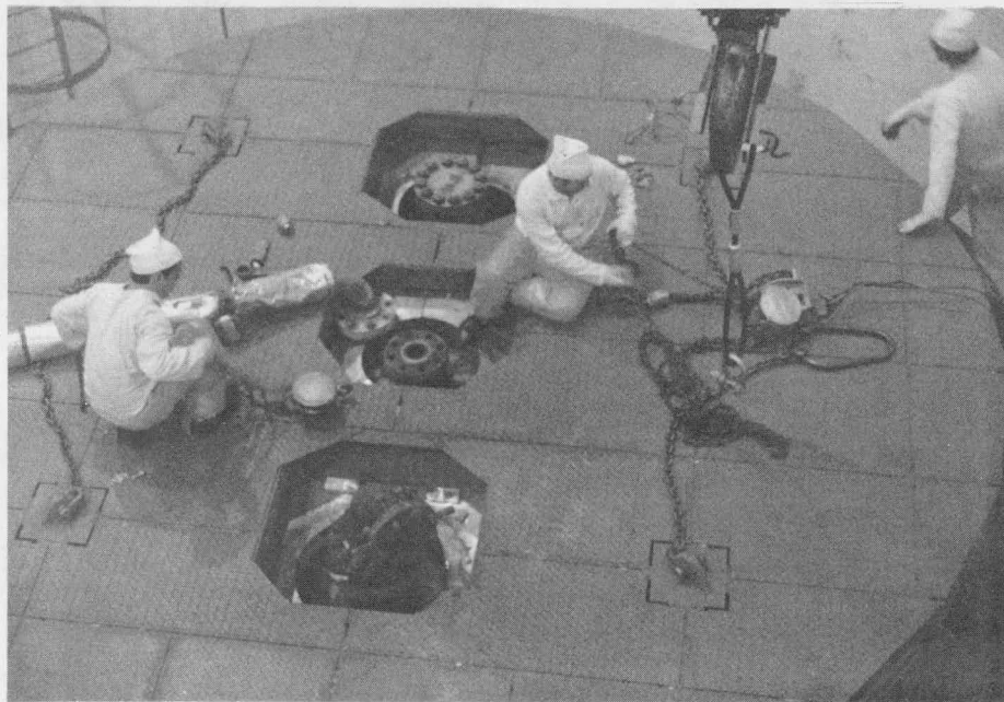
Figure 50. Rigging for Removal of Mirror Insulation (Browns Ferry)
