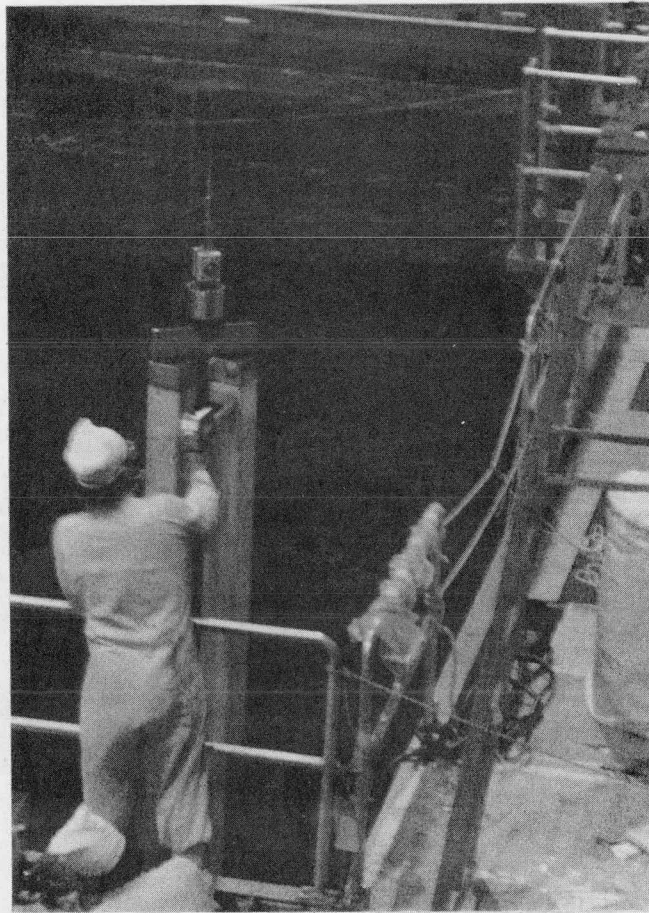
Figure 118. Health Physic Personnel using Cutie-Pie to Read Radiation of a Blade Guide (Fitzpatrick)
