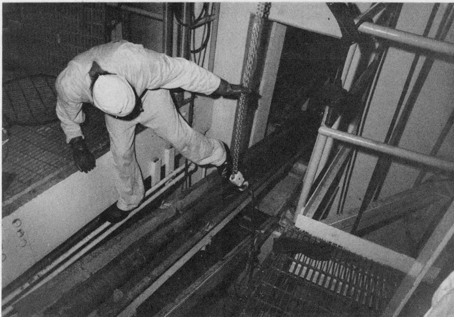
Figure 152. CRD Being Removed Freeing Binding Cable
