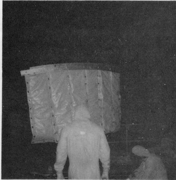
Figure 159. Reactor Pressure Vessel Temporary Shielding
