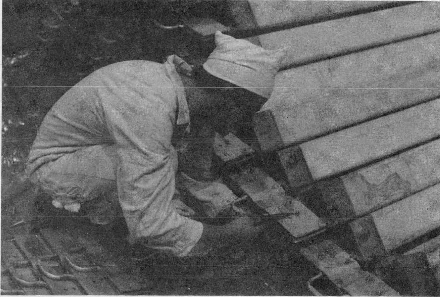
Figure 123. Attaching Brackets to Blade Guides (Fitzpatrick)
