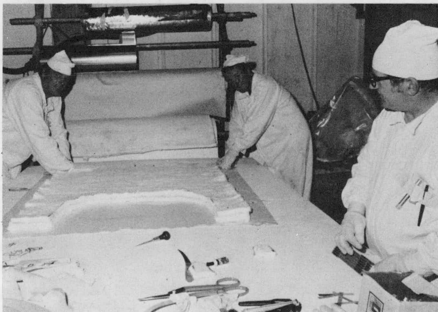
Figure 228. Cutting Drywell Piping Insulation (Fitzpatrick)
