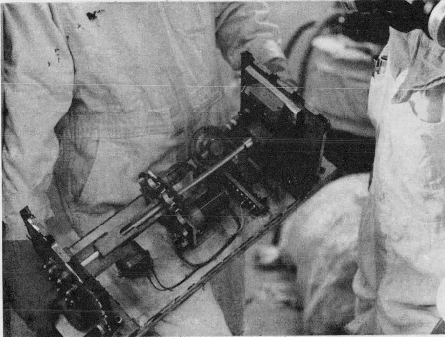
Figure 174. TIP Indexing Mechanism (Browns Ferry)
