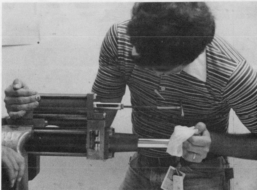
Figure 218. Reassembling Hydraulic Snubber (Browns Ferry)
