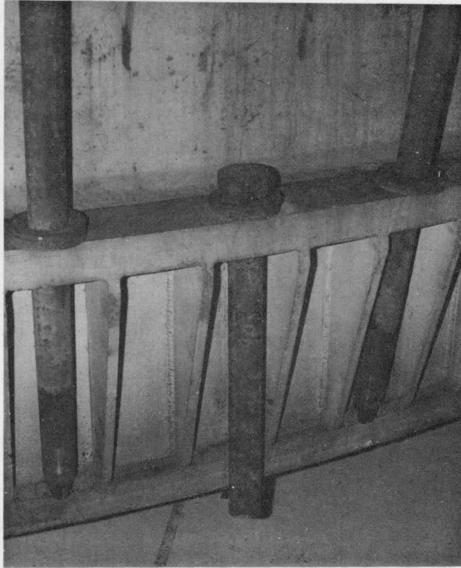
Figure 40. Corroded and Broken Drywell Head Bolts (Quad Cities)
