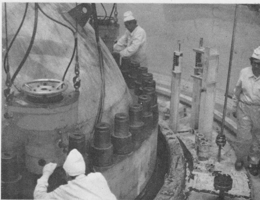
Figure 61. Head Nut Removal (Browns Ferry)
