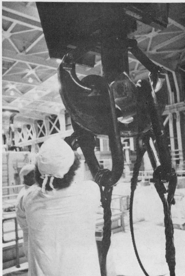
Figure 27. Rigging Inspection and Mounting for Lift - Note Center Hook Hole Used for Lifting Bail (Browns Ferry)
