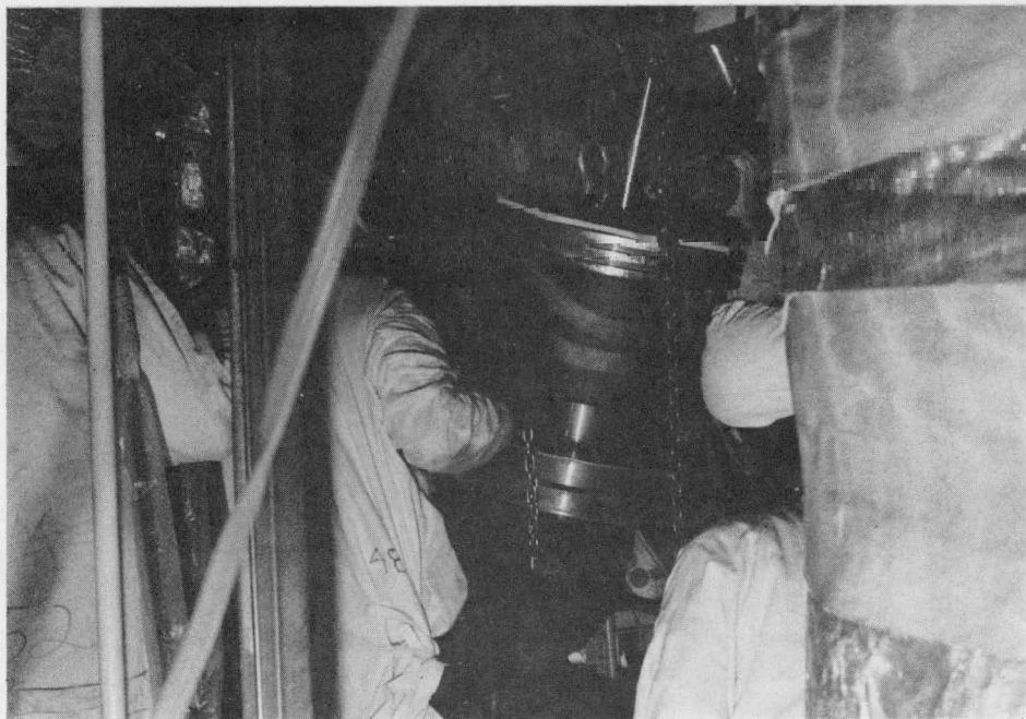
Figure 189. MSIV Internals Being Removed - Rockwell (Fitzpatrick)
