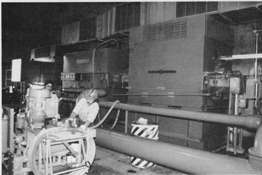
Figure 241. Adding Hydraulic Fluid to M. G. Set (Fitzpatrick)
