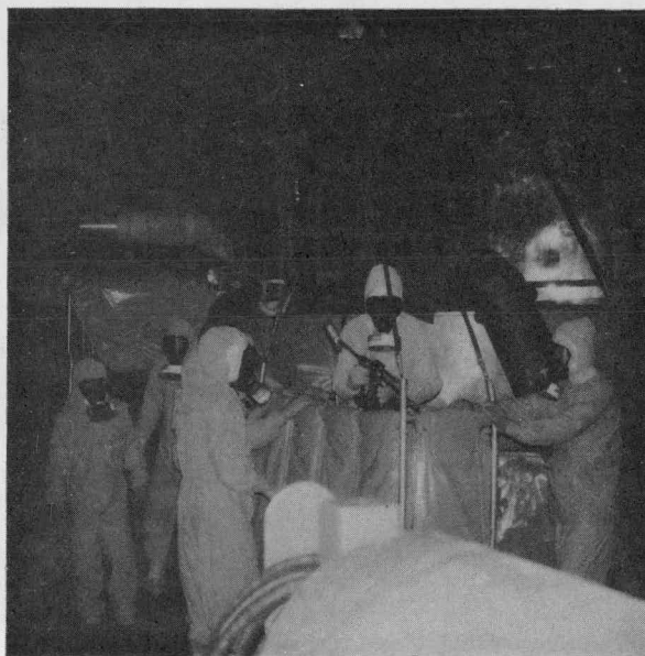
Figure 96. Personnel in Crane Skip Preparing to Hydrolase Reactor Cavity
