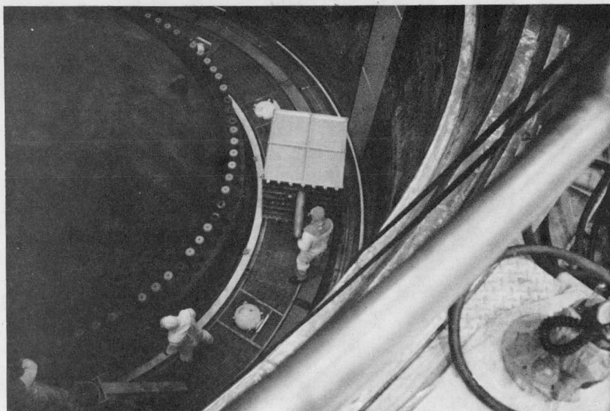
Figure 64. Installing Head Bolt Thread Shield Cylinders (Browns Ferry)
