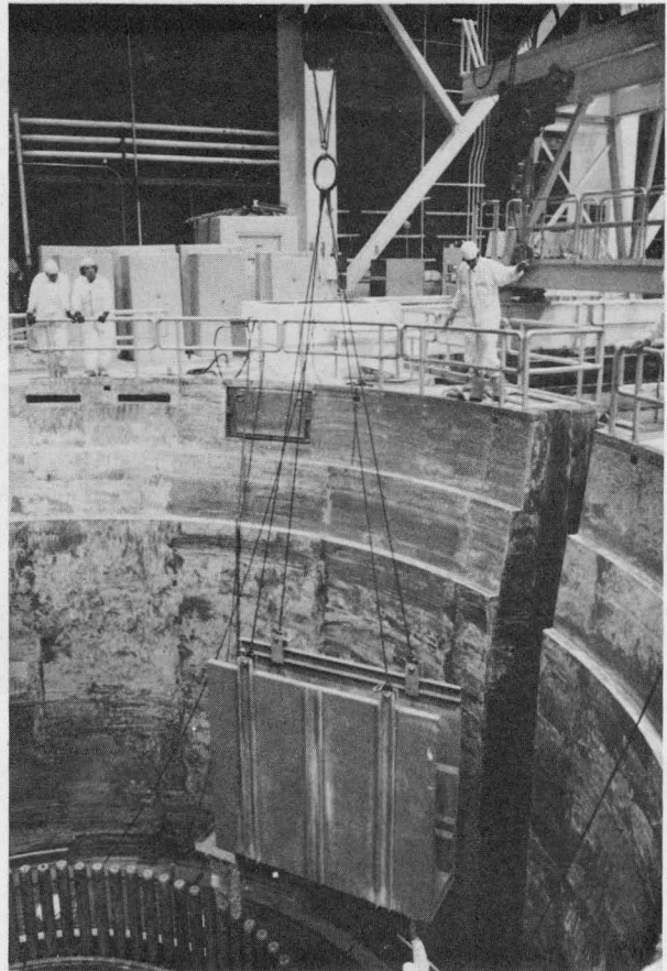
Figure 102. Installing Cattle Chute into Refueling Slot - Main Crane Being Used (Browns Ferry)
