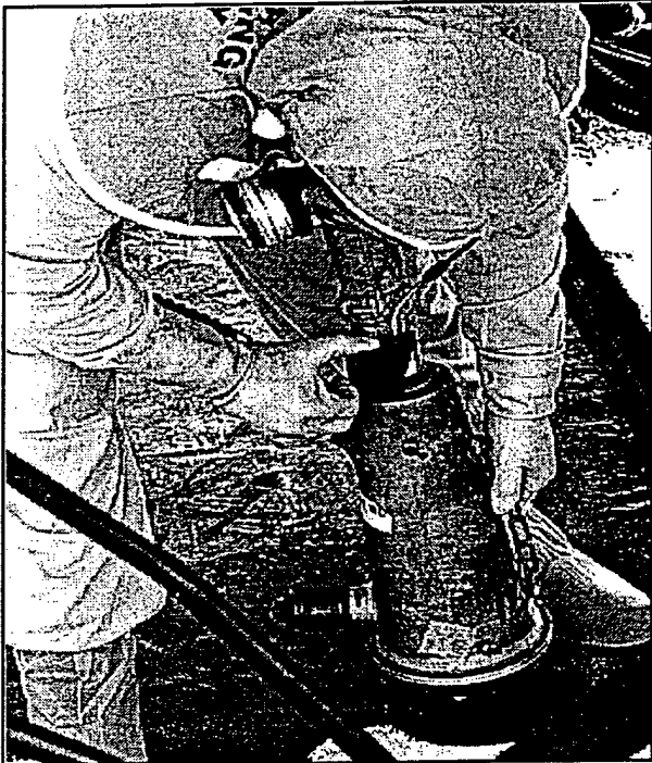
Figure 1- Manual operation of shotblast head.
