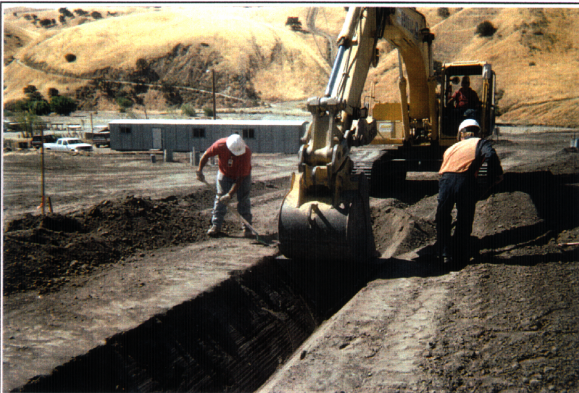
Photo 14: Cutting concrete lined V-ditch with a specially made bucket.
