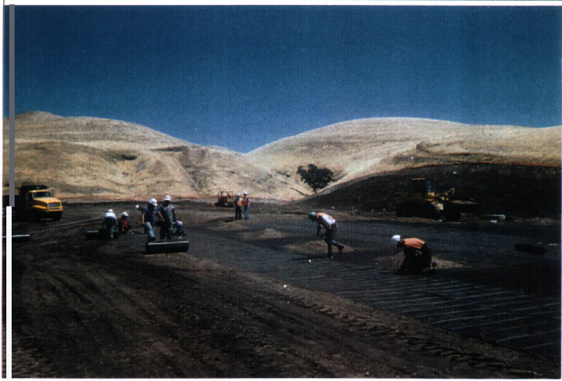
Photo 4: Installing geogrid, tying panel together with plastic zip ties every 5 feet.
