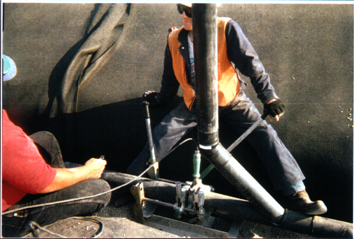
Photo 15: Welding 4-inch SDR-17 HDPE pipe in drainage ditches over drainage rock
