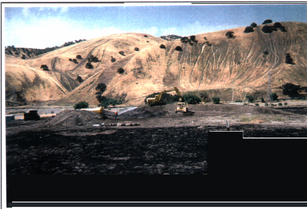
Photo 2: Preparing subgrade by pushing soil berms into landfill with CAT 650LGP.
