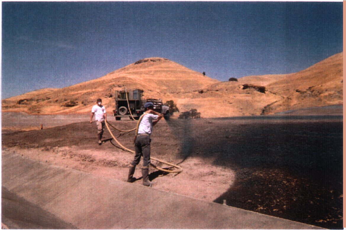
Photo 18: Spray application of hydroseed over landfill area.
