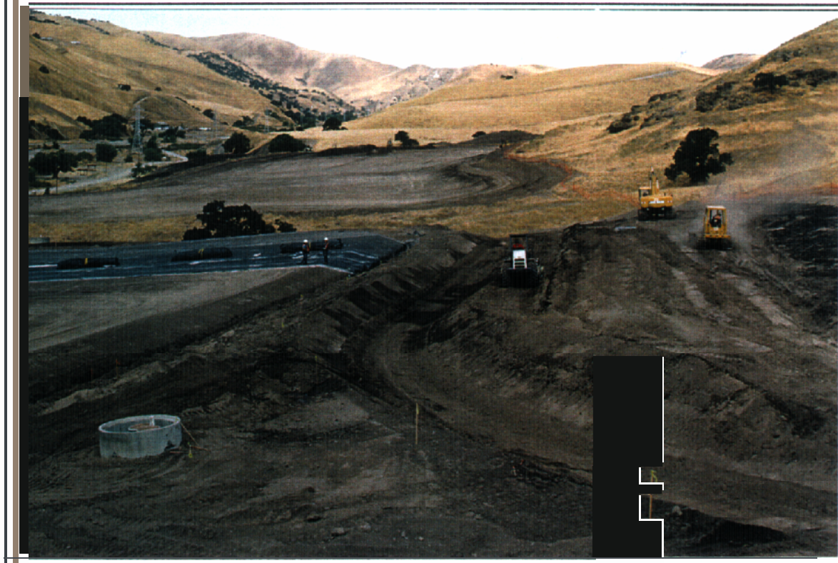
Photo :7 Replacement and compaction of north berm fill.
