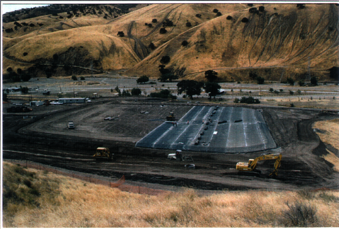
Photo 8: Deployment of GundSeal® over general fill. Working on north diversion ditch.
