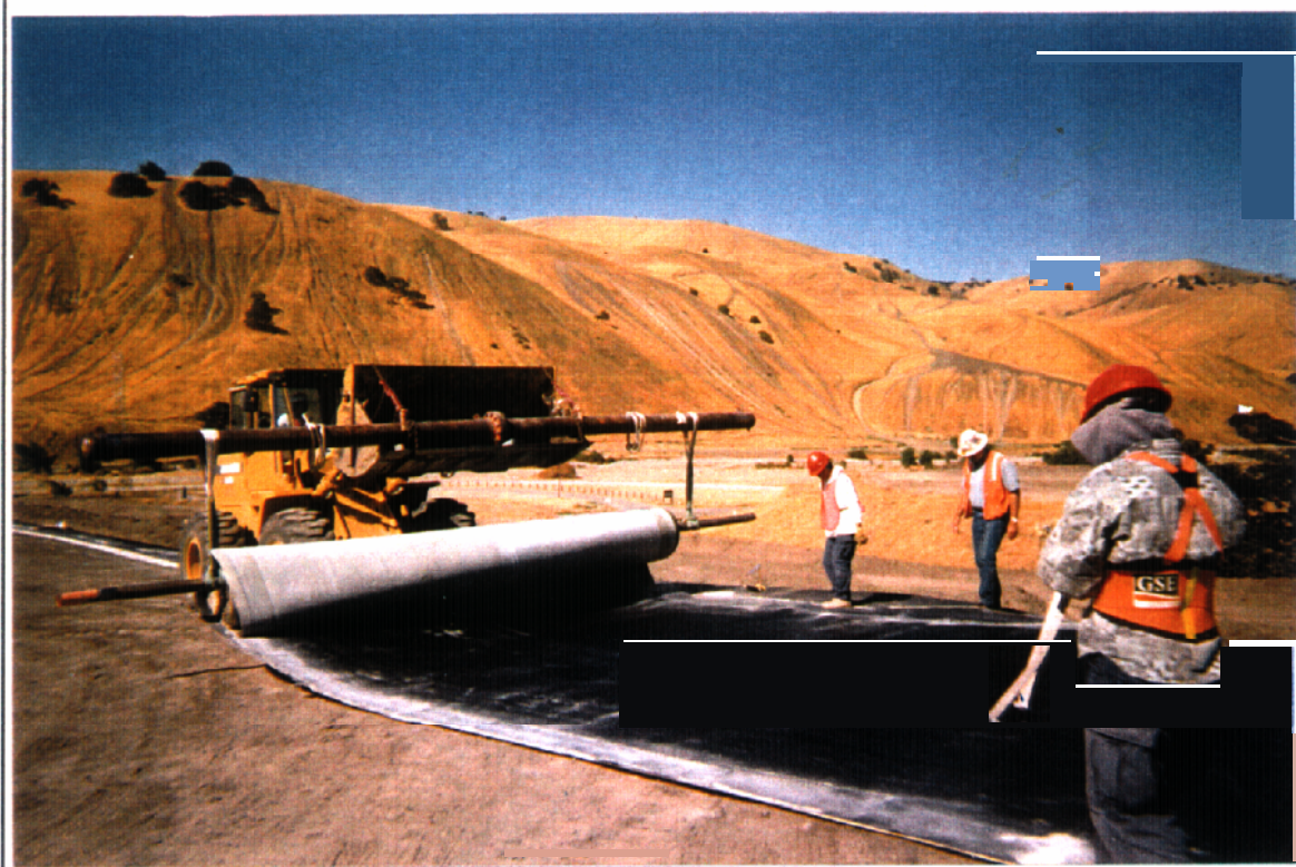
Photo 5: Deployment of GundSeal® over prepared general till.
