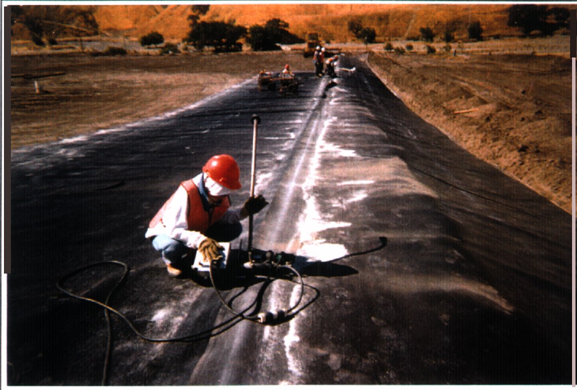
Photo 6: Fusion welding of GundSeal® panels with a wedge welder.
