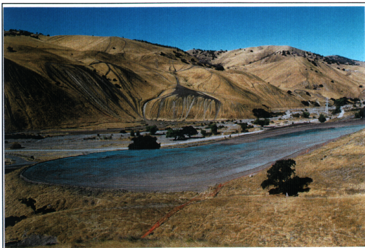
Photo 20: Hydroseeding on soil borrow area
