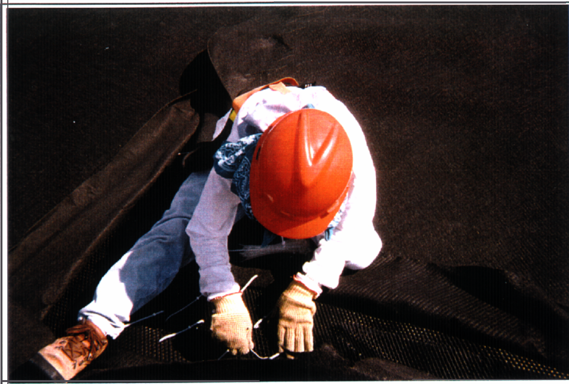
Photo 11: Tying geocomposite at but seams, two rows at 6-inches staggered.
