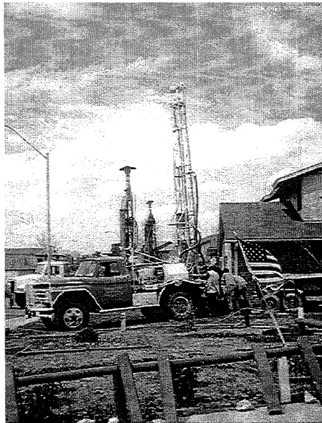
Fig. 1.4. A rig drilling vertical boreholes for the ground heat exchangers. A total of 1,834,652 ft of 4 1/8-in. vertical bore was drilled for the vertical borehole heat exchangers.
