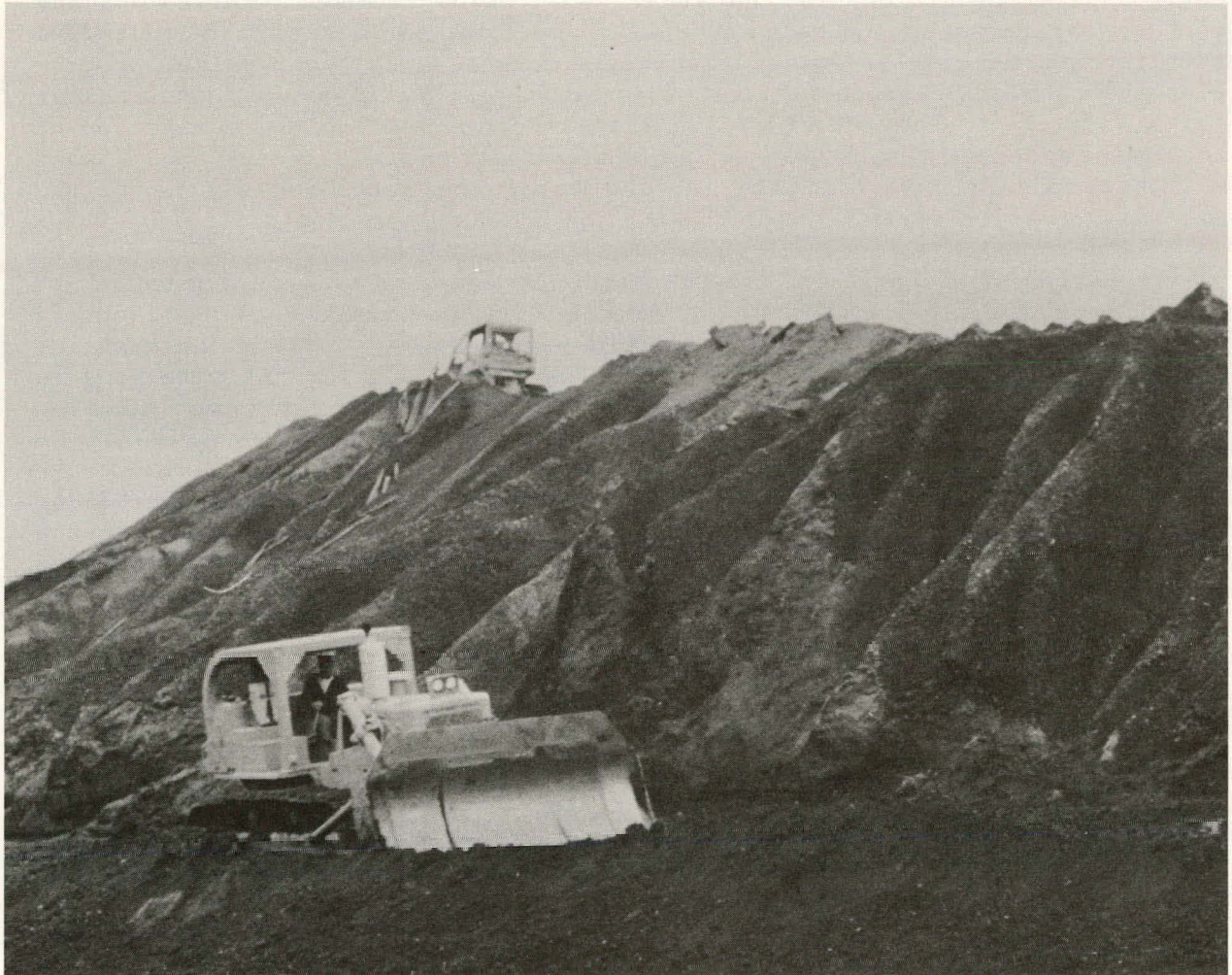
Fig. 3. Rough Grading the Gob Pile Early in the Site Development Phase
