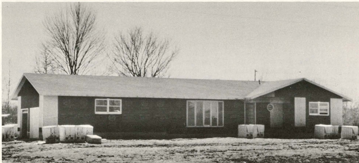
Fig. 14. Home Under Construction Near the Staunton 1 Site
