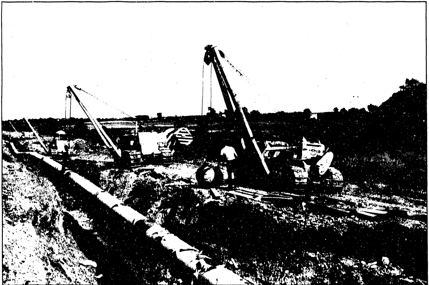
Natural gas pipeline being lowered into trench. Photo courtesy: Bob Thigpen, Texas Eastern Transmission Corp.
