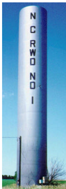
Figure 4.16 Rural Water District standpipe (Nemaha County).
