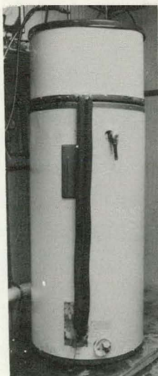
Figure 3-3 Unit Showing Refrigerant Lines on Side.
