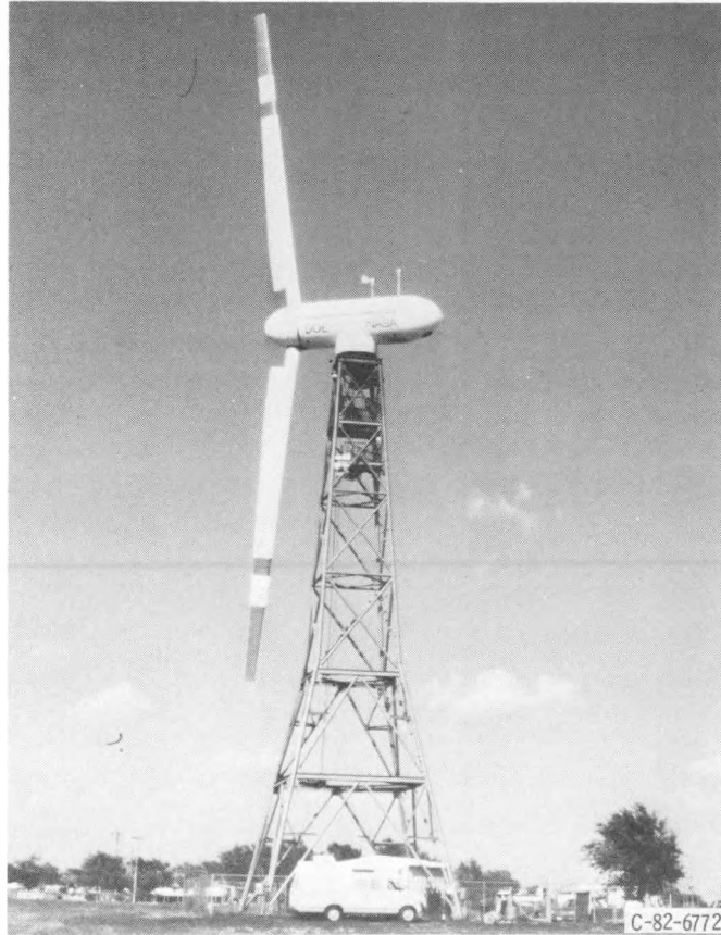
Figure 1. - 200-kW Mod-0A wind turbine with SCI fiberglass blades at Clayton, NM.
