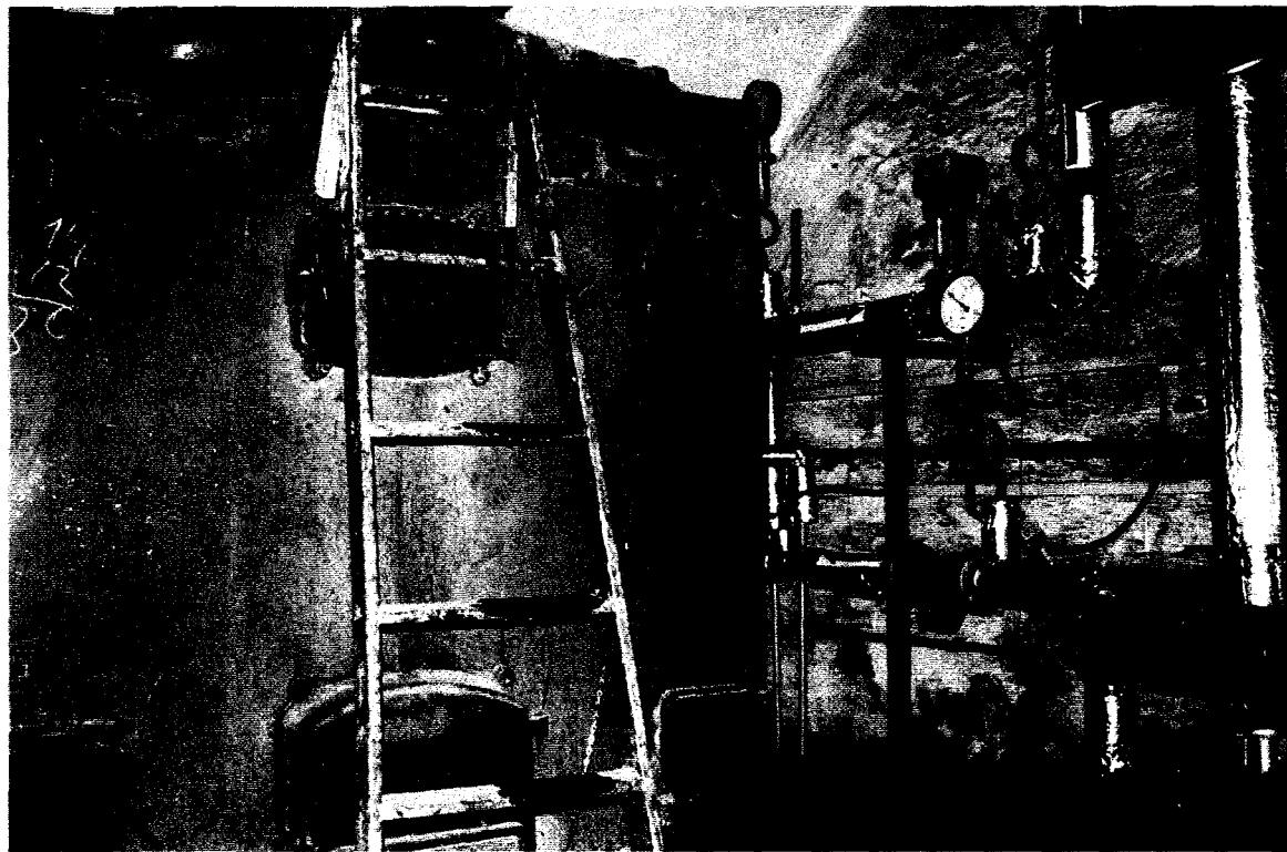
▲ Recently retired boiler and new heat exchanger at Szeroka 35
