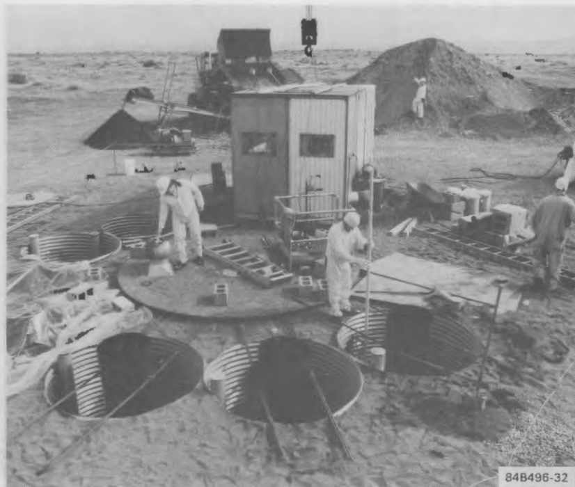
FIGURE 9. Construction Site Showing Sleeves in Empty Lysimeters
