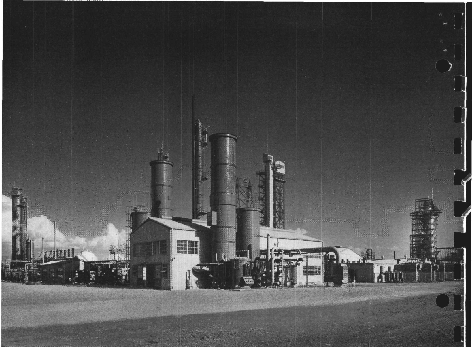
Air, water and natural gas are converted into ammonia and urea in this chemical plant designed and constructed by Foster Wheeler Corporation.
