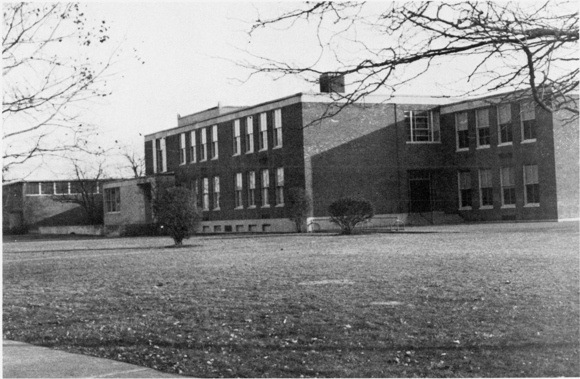
FIG.3-2 NORTH FACE ORIGINAL BUILDING
