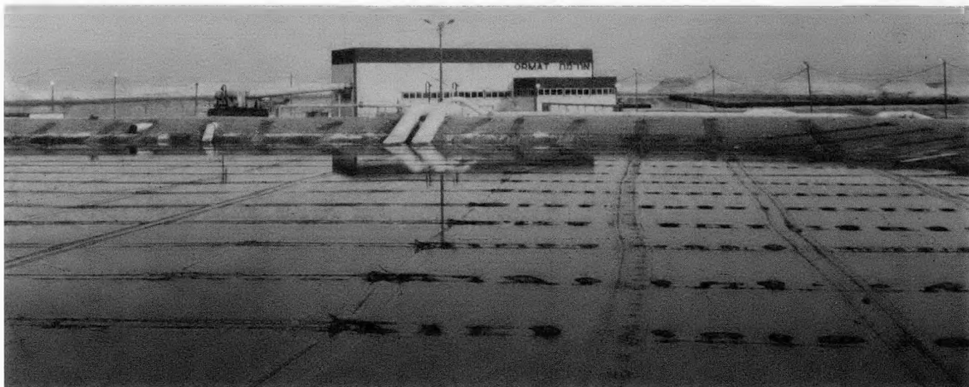
5-MW Solar Pond Facility at Beit Ha'arava, Israel
