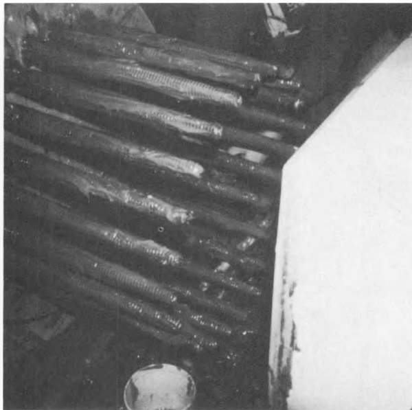
Figure 55. - Application of thickened adhesive to studs.
