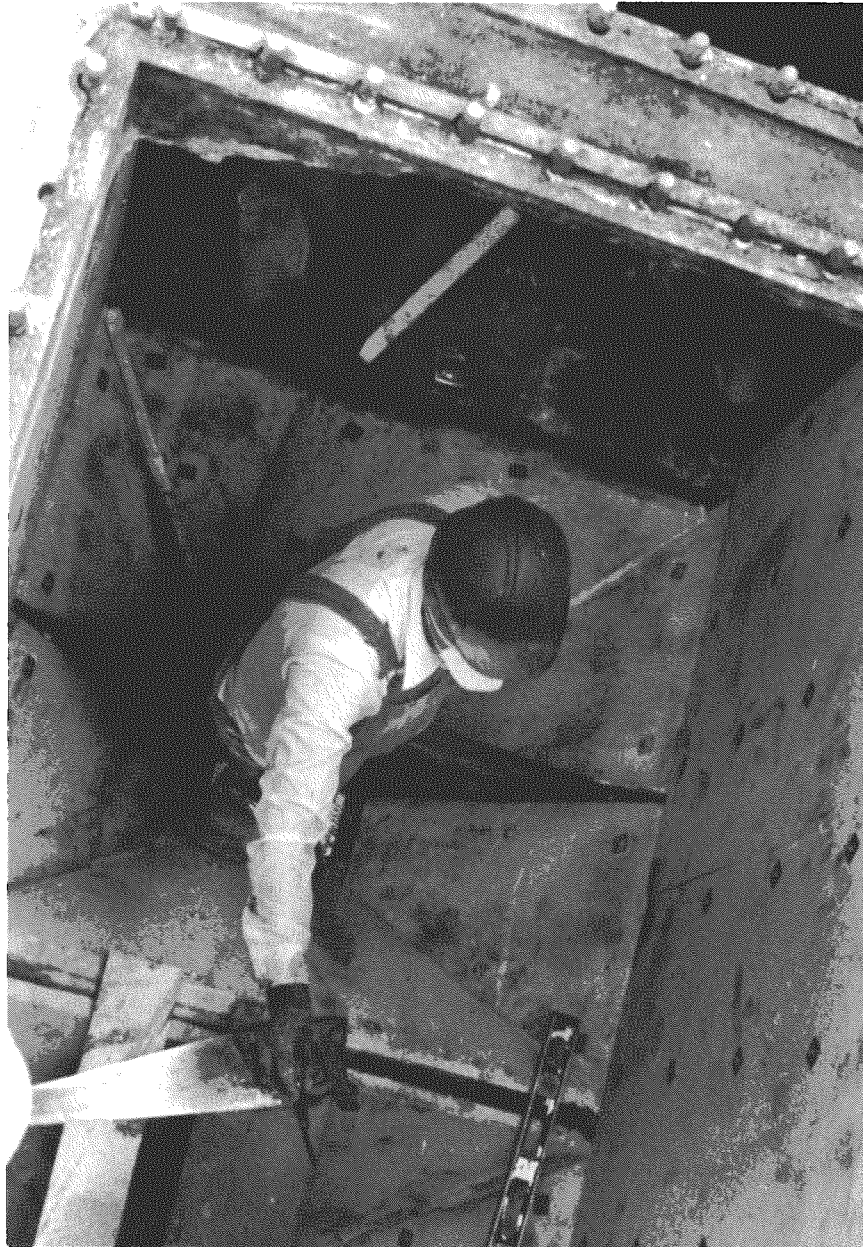
Figure 6. Installation of Aluminosilicate Fiber Refractory in SHTM
