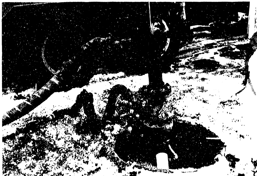
Fig. E-8. Close-up of well configuration. A 12.5-cm hose is a water line to kill the well, and a 6.0-cm pipe carries the cement.
