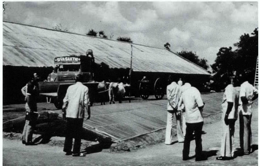
This solar rice dryer in Nepal can handle 75 tons of rice per day, and has been operating since 1984.
