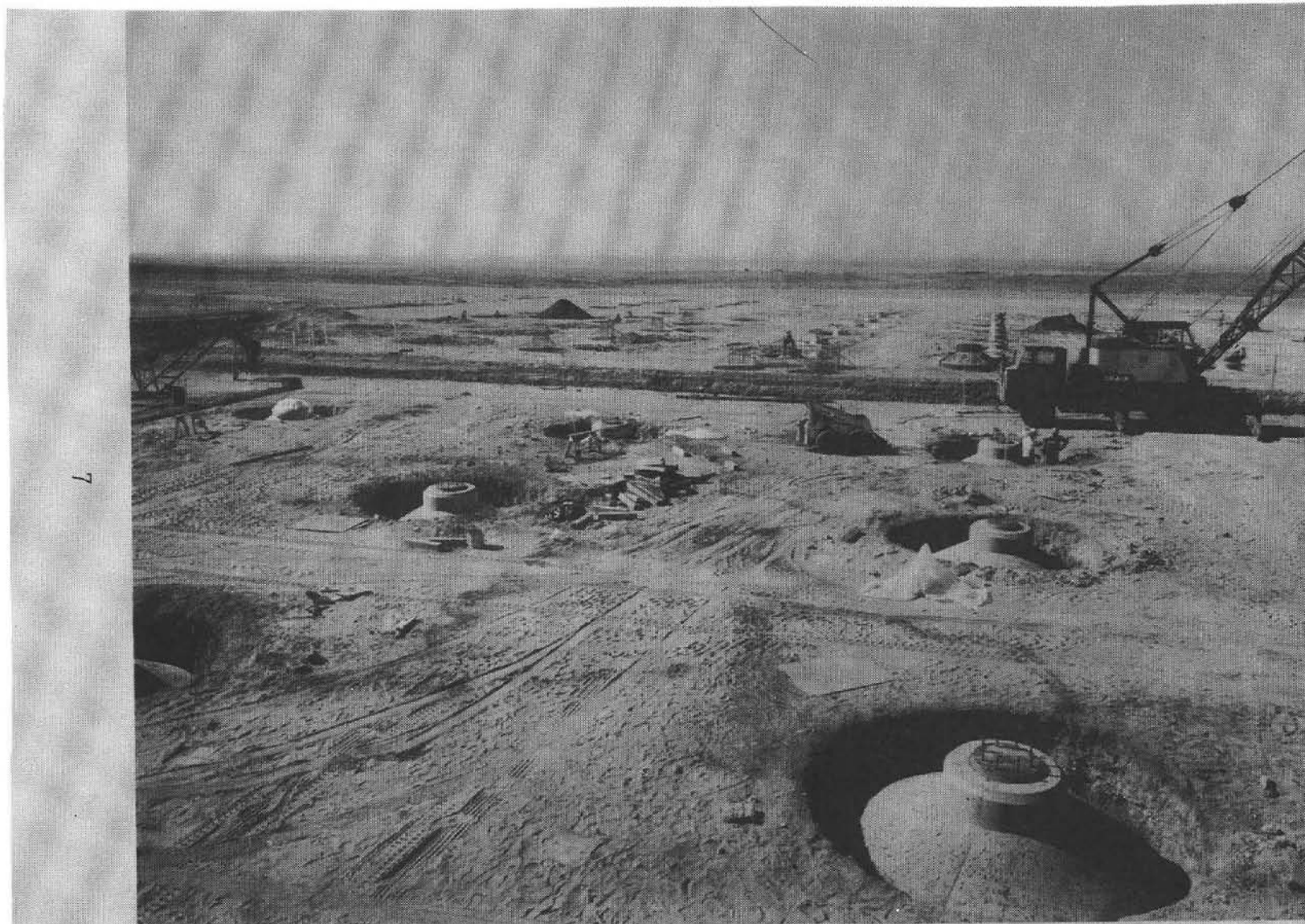
HELIOSTAT FOUNDATION INSTALLATION
