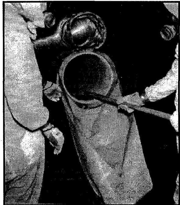
Figure 8. Deposit Removal Using Standard Decontamination Tools (Shovels, Hoes, Chisels)
