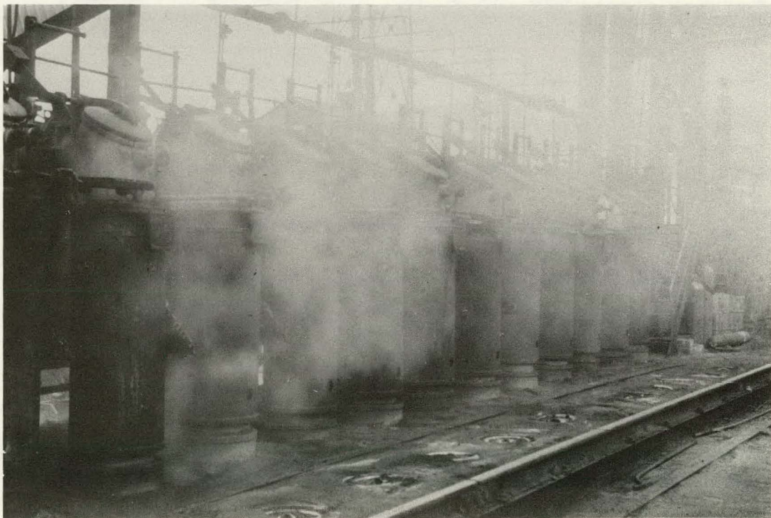
Fig. 8. Ascension pipes with leaking vapours.
