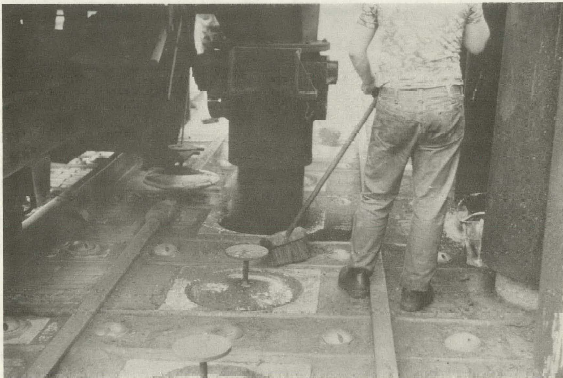
Fig. 4. Charging procedure for coke oven.
