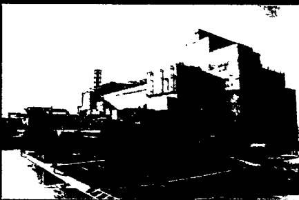
The Defense Waste Processing Facility immobilizes waste by turning it into glass logs. The process, called vitrification, adds glass-forming materials to the waste, heats the mixture in a melter, and pours the molten glass into canisters.
