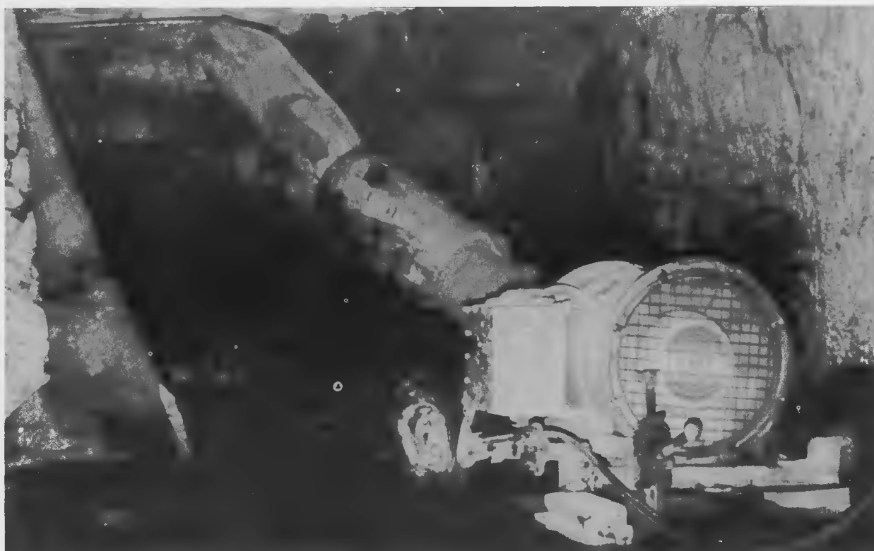
FIGURE 4. - Face ventilation system employing blowing tubing behind a blowing line brattice.
