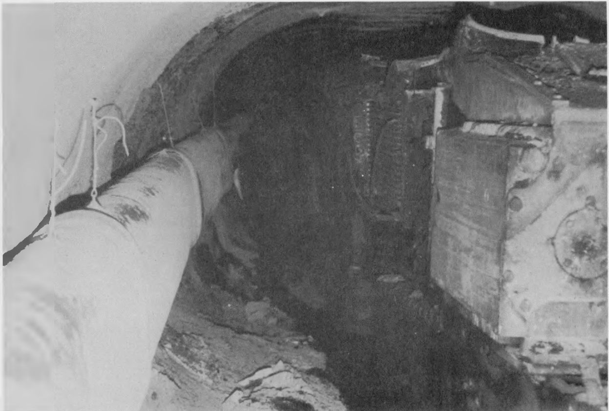
FIGURE 7. - Elliptically shaped fiberglass tubing employed on a boring machine section.
