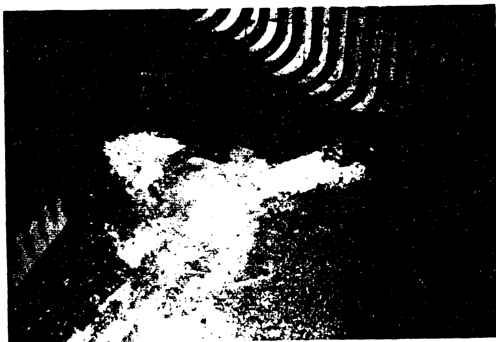
Figure A-III-32: Photo of rear boiler floor and lower boiler tubes taken at the same time as figure A-III-30. Note the high ash/char deposits in right rear corner of boiler. June 1988.
