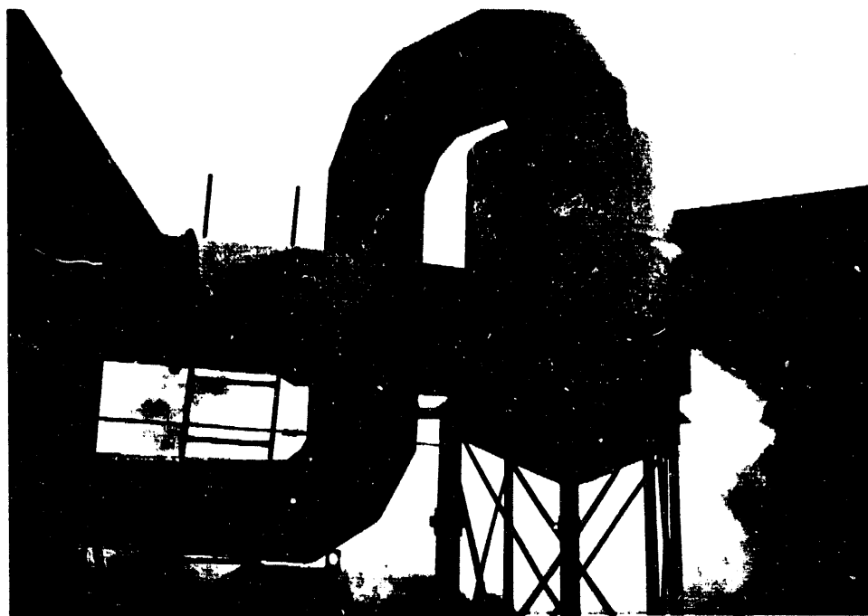
Figure A-III-46: Scrubber fan with its stack, as well as connecting duct from scrubber vessel to fan installed on roof of boilerhouse. The steam flow-off silencer is at lower right. Summer 1987.
