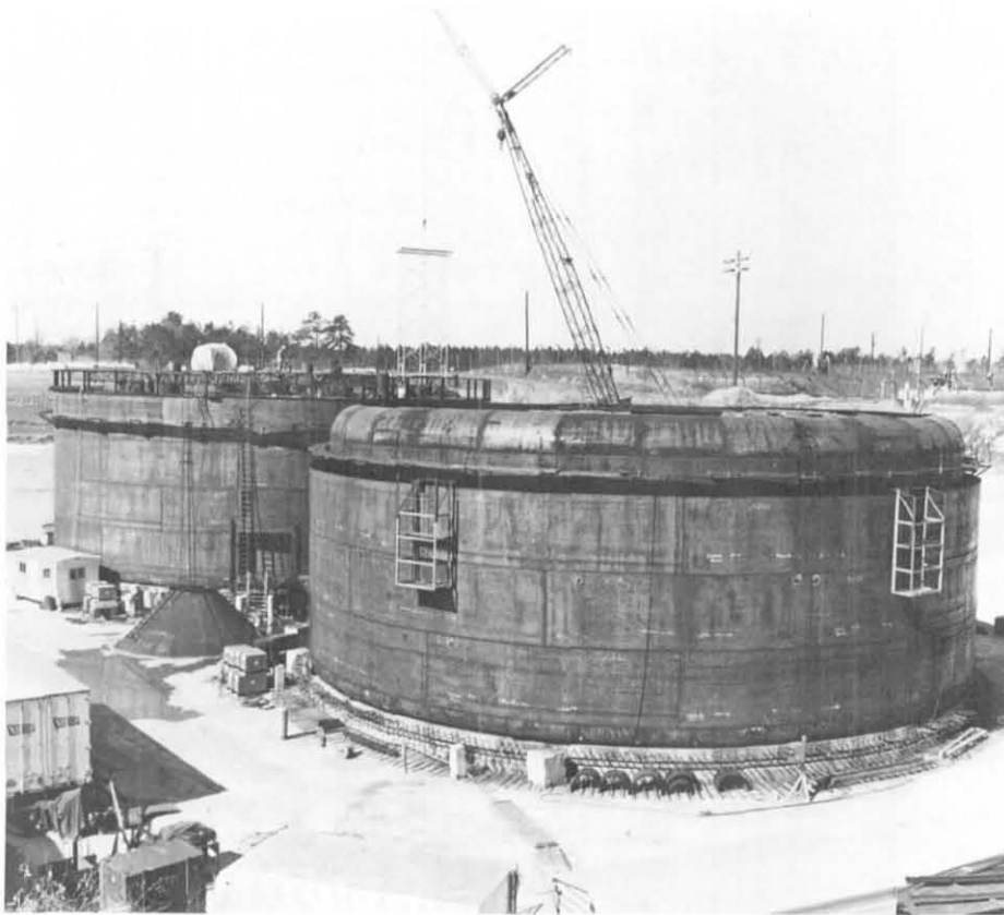
High-level waste storage tanks. . . The 30 high-level radioactive waste storage tanks at the Atomic Energy Commission's Savannah River Plant in South Carolina were built of carbon steel, surrounded by concrete encasements two to three feet thick, set about 40 feet in the ground and back-covered with dirt. Each had a capacity of from 750,000 to 1,300,000 gallons. Most tanks were equipped with cooling coil assemblies to remove heat produced by radioactive decay of fission products in the waste. Pictured here are two steel tanks before concrete encasement. They consist of a tank within a tank. The outer liner on the tank in the background is finished. The rounded, inner primary steel liner is visible at the top of the tank in the foreground.
