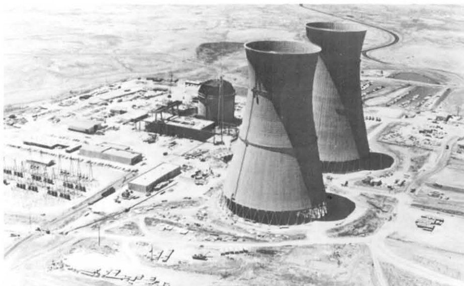
Rancho Seco Nuclear Station. . . These twin hyperbolic cooling towers, 43 stories tall, are an integral part of the plant developed by the Bechtel Corporation at the 913-Mwe. Rancho Seco Nuclear Station in California. Located 25 miles southeast of Sacramento, the plant was constructed for the Sacramento Municipal Utility District. The natural draft evaporative towers dissipate waste heat by recirculating the turbine condenser cooling water on a gigantic scale—a half million gallons per minute.
