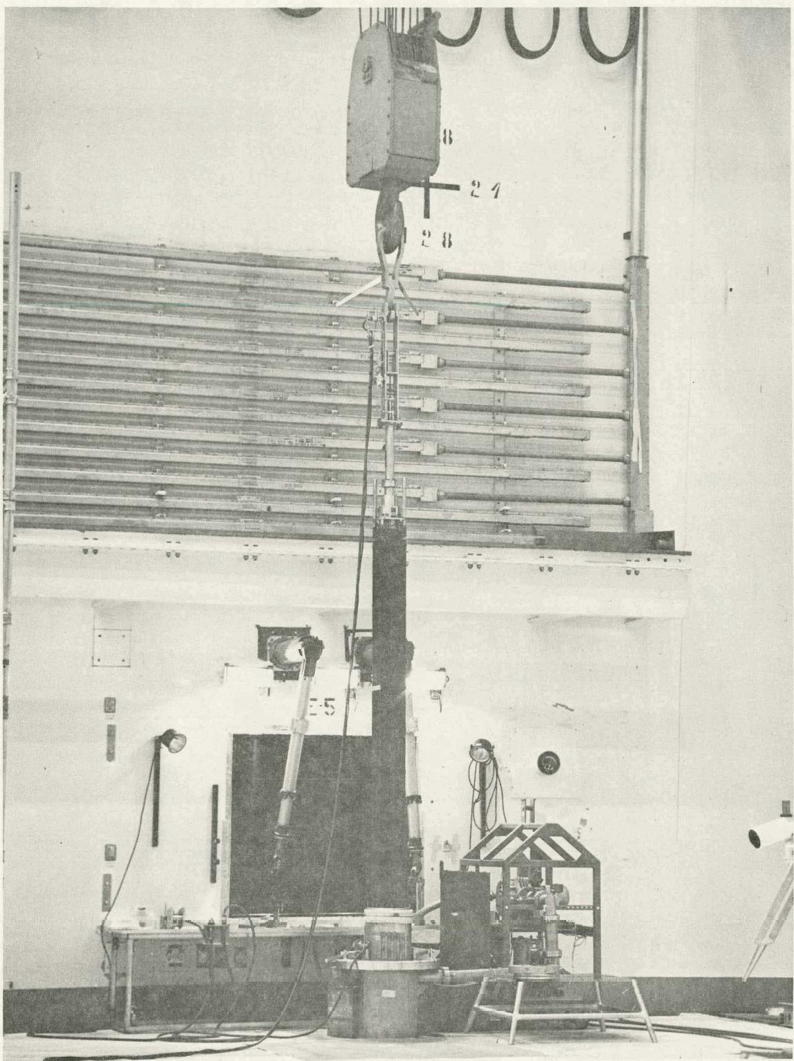
Figure A-8. PWR Fuel Assembly Being Installed Into Canister
