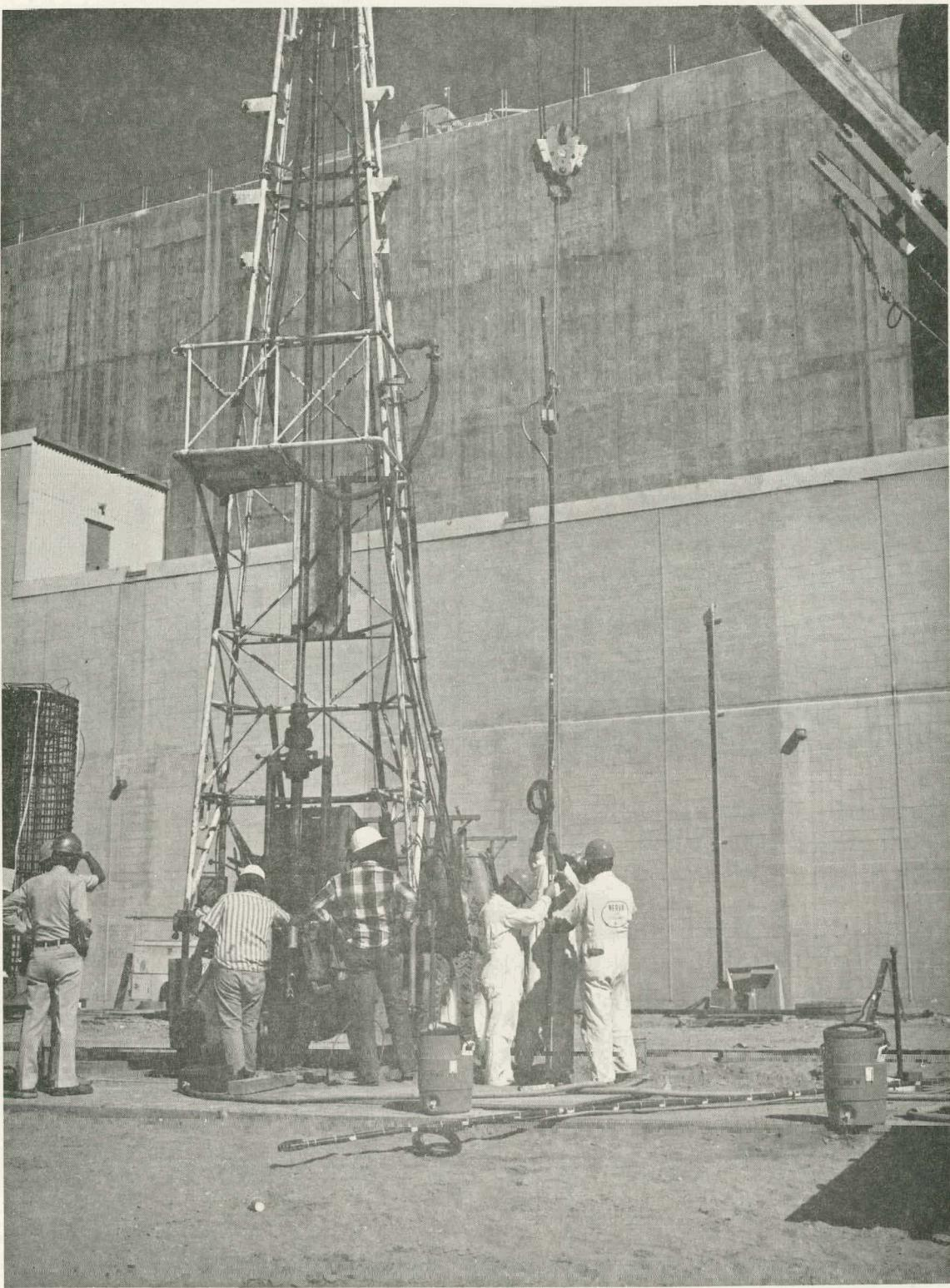
Figure A-6. Instrumentation Well Installation
