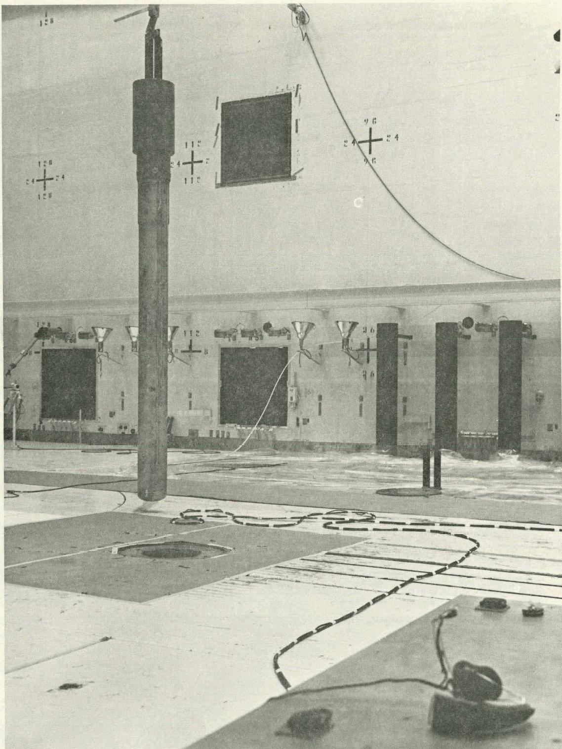
Figure A-9. Placing Completed Canister Assembly in Hot Bay Transfer Pit
