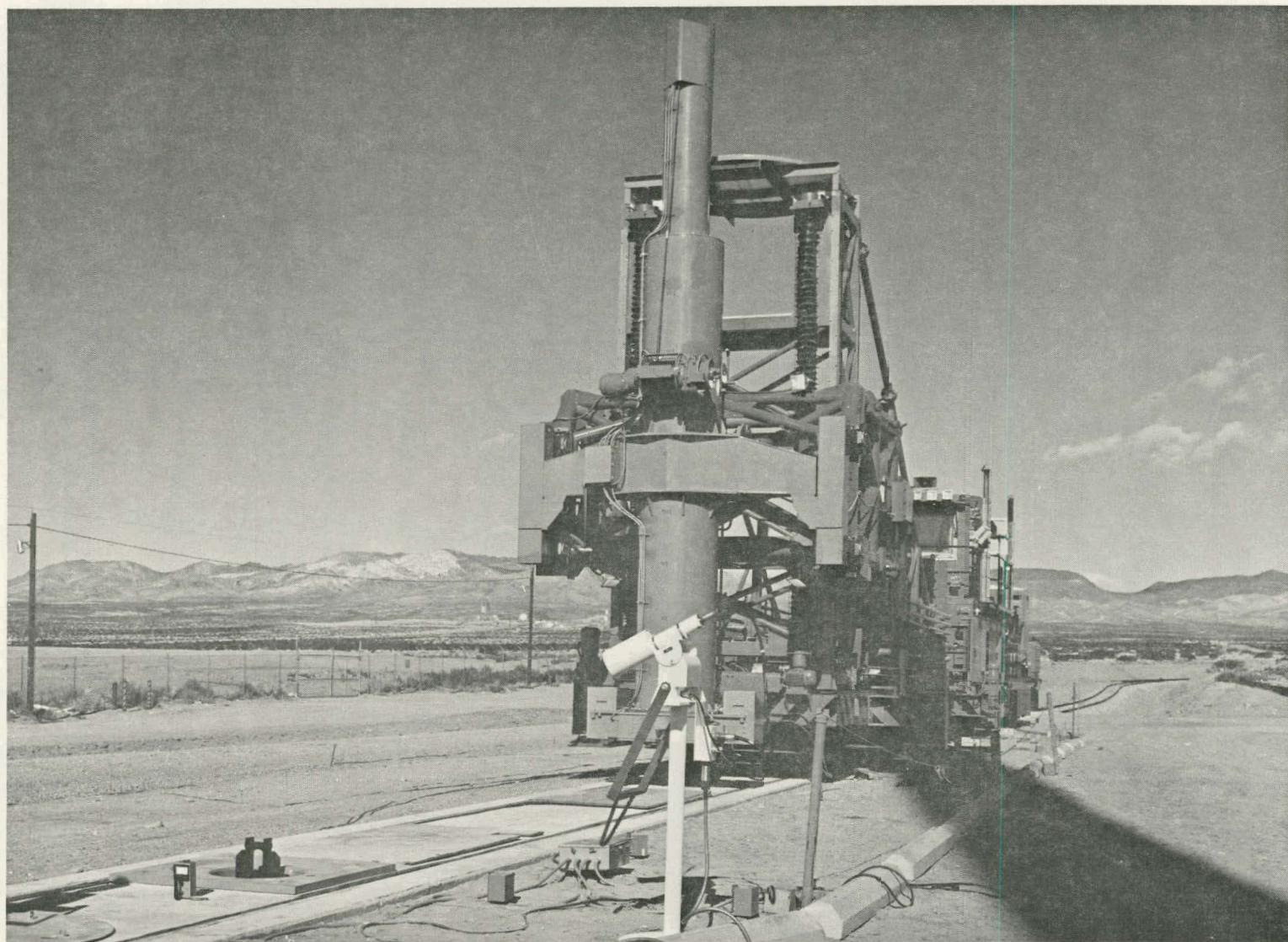
Figure A-12. Transfer of Canister to Drywell Completed
