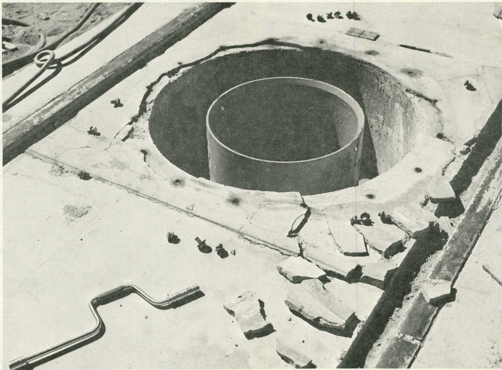
Figure A-17. Drywell 5 at End of Isolated Drywell Test With Cover Plate and Canister Removed
