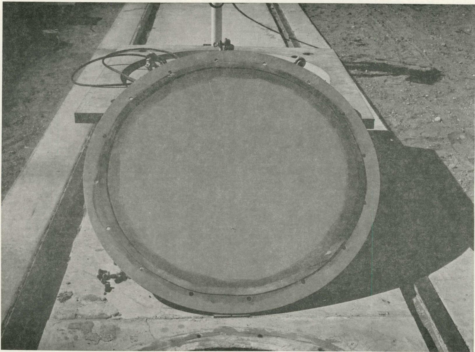
Figure A-14. Drywell Cover Plate Showing Neoprene Gasket
