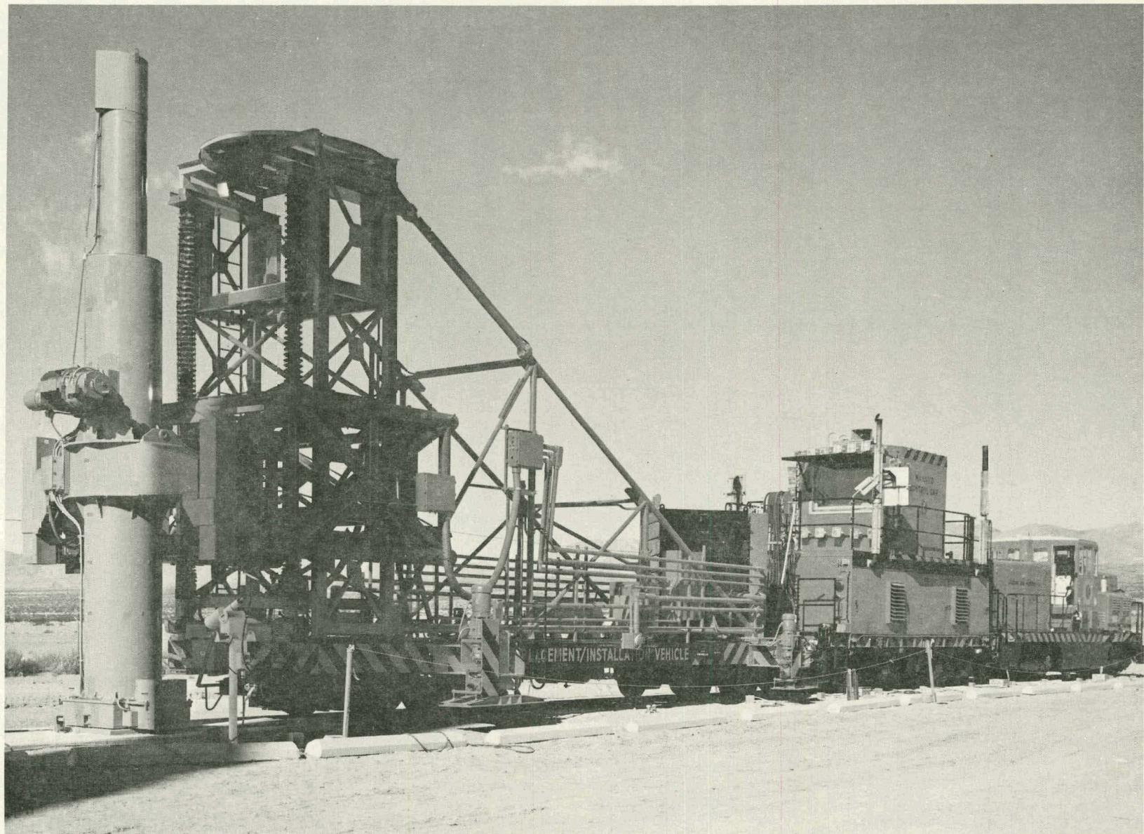
Figure A-11. Transfer Shield Positioned Over Drywell Emplacing Canister Assembly in Drywell
