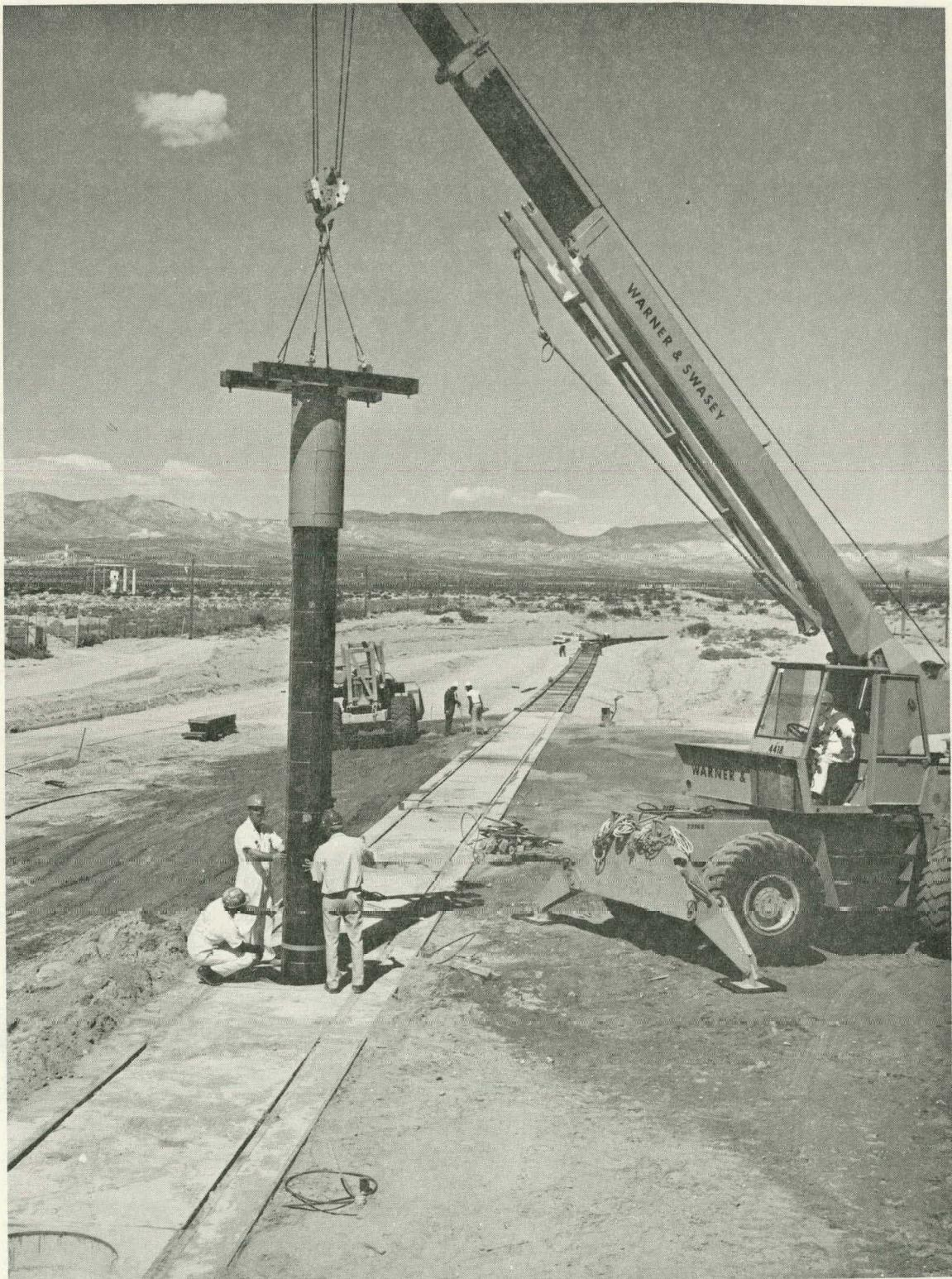
Figure A-5. Drywell Liner Installation Into Storage Area
