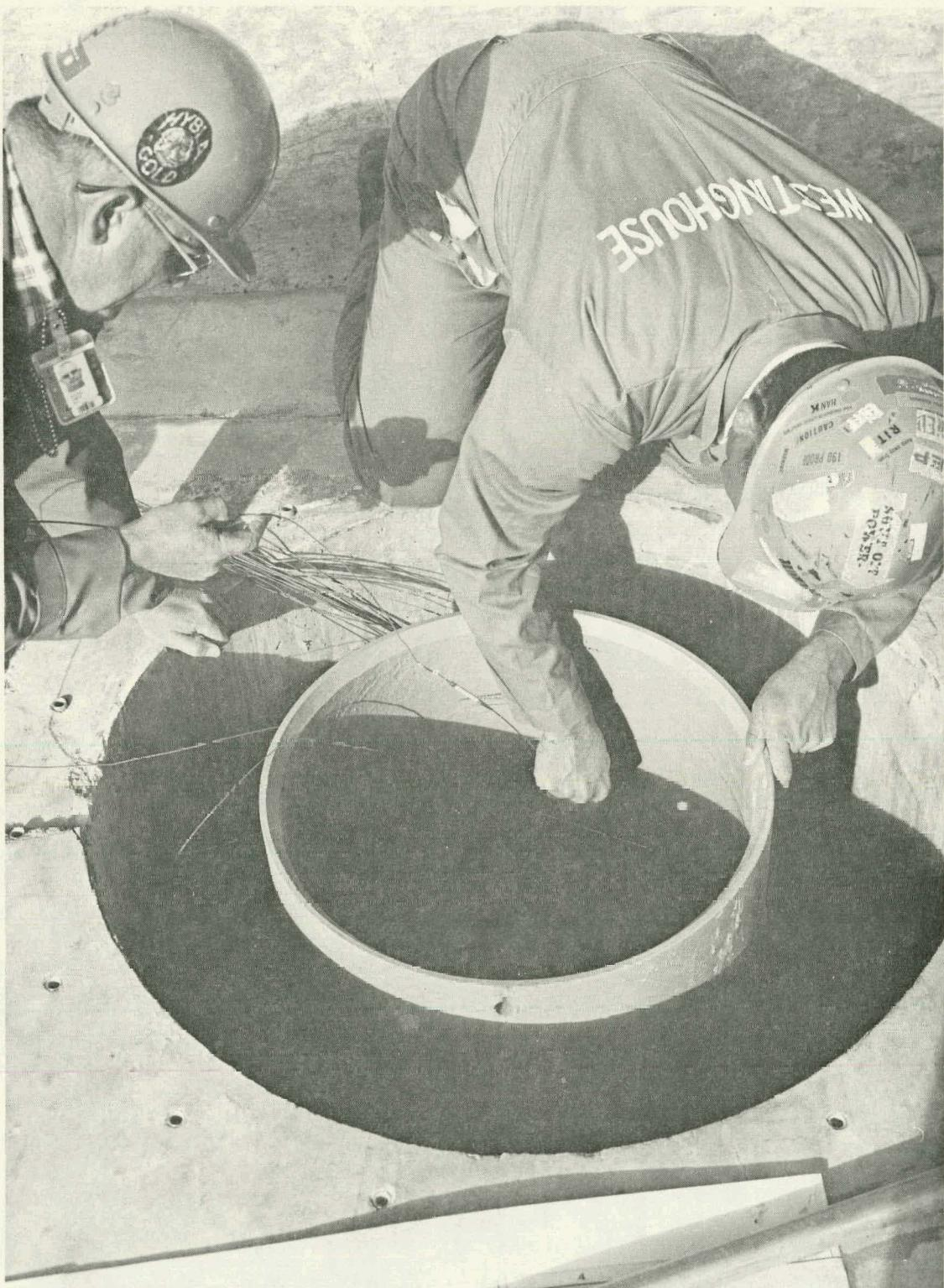
Figure A-13. Insertion of Thermocouples Into Drywell and Into Canister Through Shield Plug
