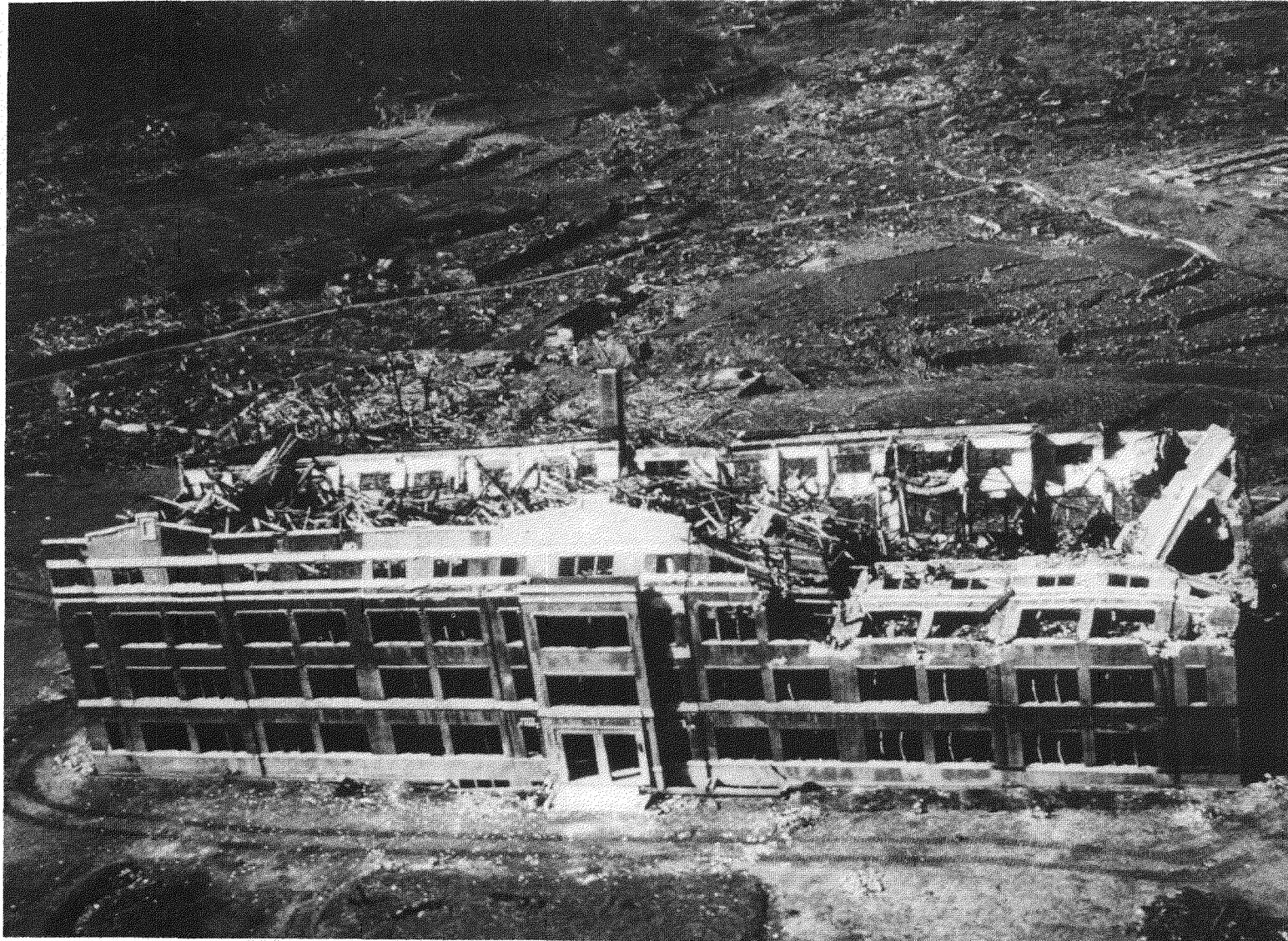
Fig. 12. Reinforced concrete building in Nagasaki (Chinzei School, used as a factory machine shop).
