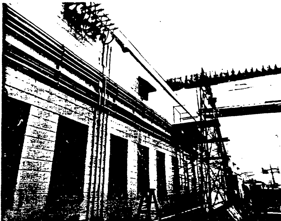
Figure 3. Scaffolding for Ductwork Replacement.
