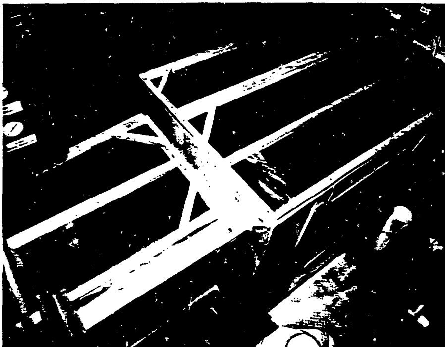
Figure 4. Typical Containment Tent for Hot Work.
