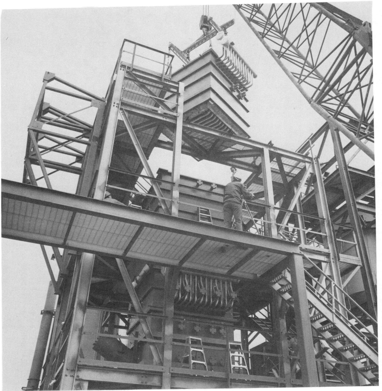
Figure C-20. Convection Section Being Installed in Platform
