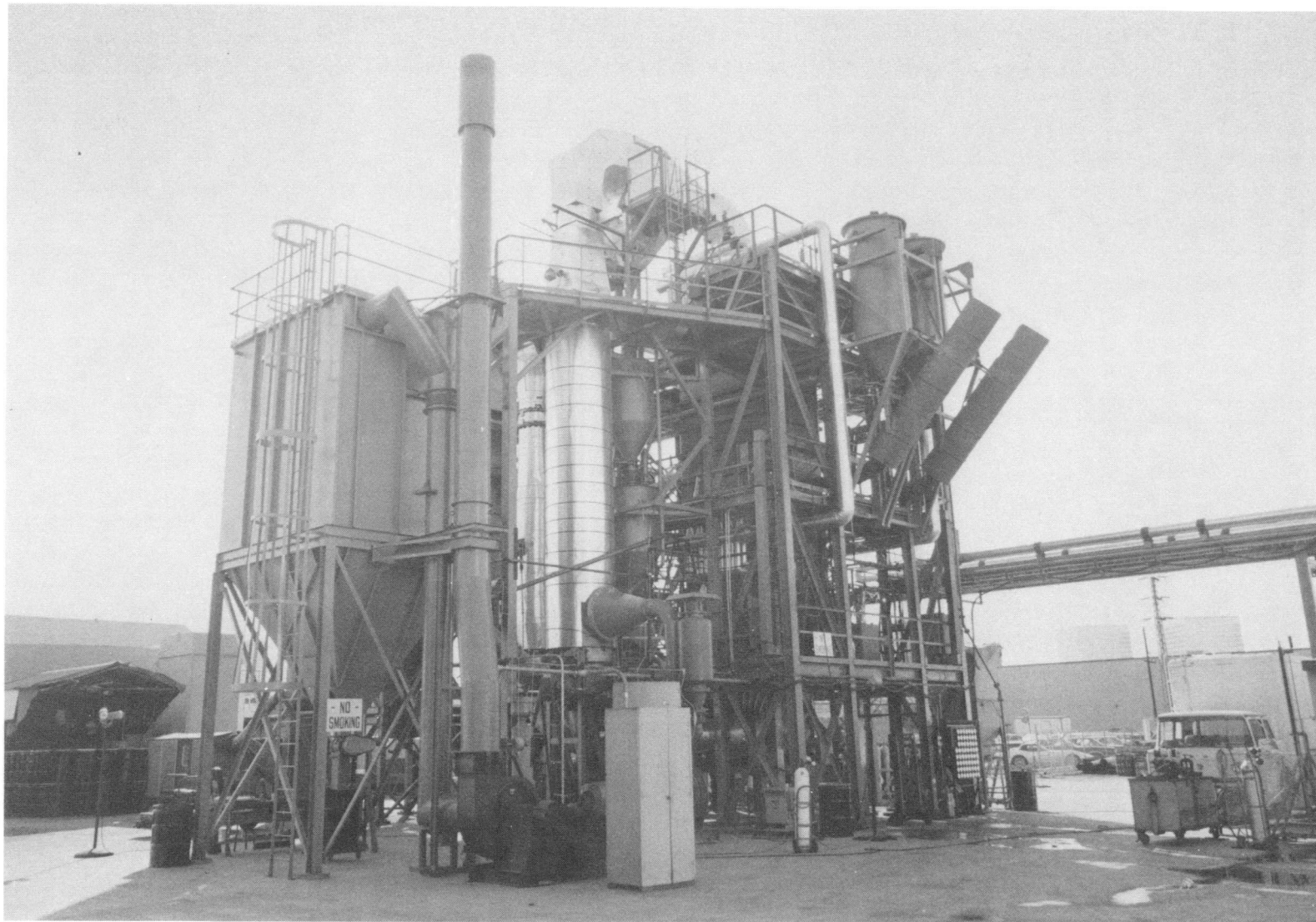
Figure C-3. Overall Facility - North and East Elevations (left to right, baghouse, exhaust stack, air preheater, ash recycle bins, and combustor/heater in main platform; upper right of platform are the limestone and spent bed material bins, and the working fluid mufflers)
