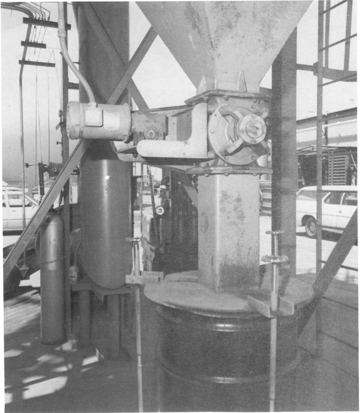
Figure C-62. Baghouse Drain (periodically, the baghouse was drained into drums used for disposal)
