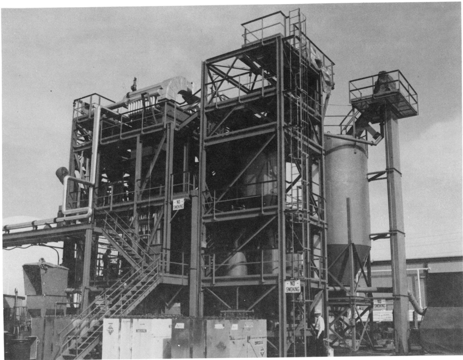
Figure C-2. Overall Facility - West Elevation (main platform and coal tower; working fluid air supply tressel at middle left, limestone fill station at lower left)
