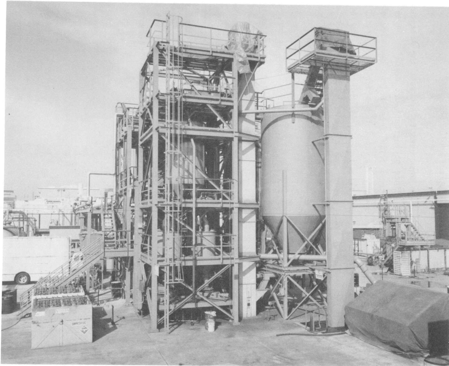
Figure C-1. Overall Facility - South Elevation (in the foreground are the coal tower, coal silo, and coal receiving pit)
