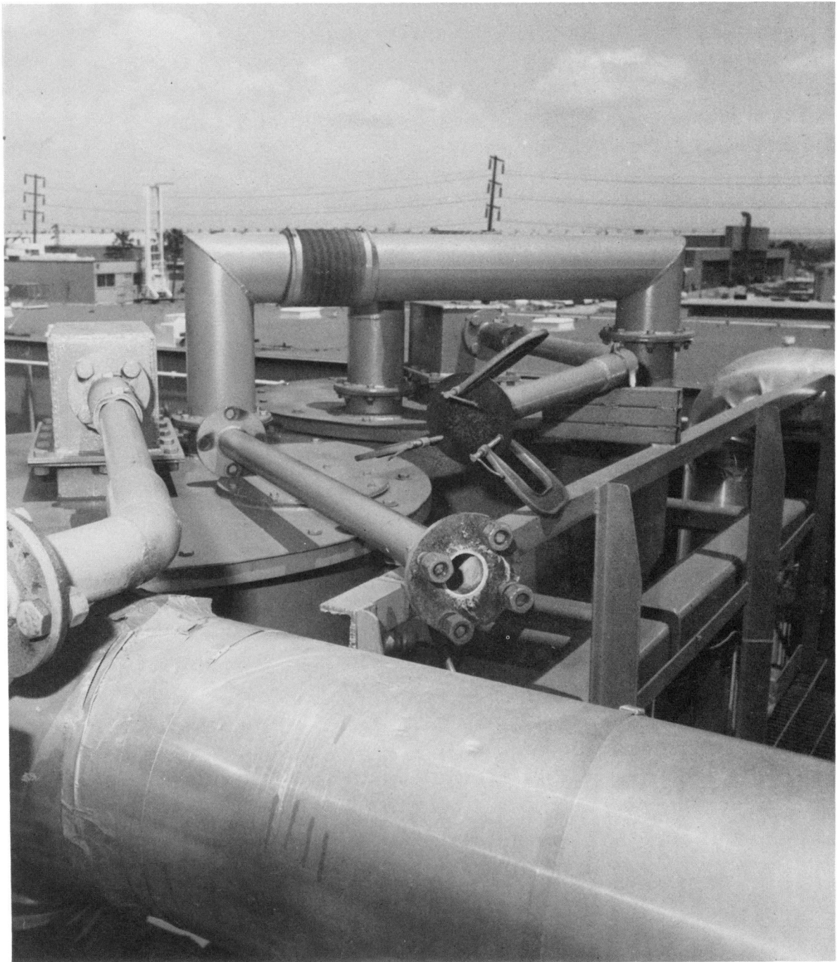
Figure C-64. Top of Limestone and Spent Bed Material Bins (lines were changed to allow the limestone fill station to be used to fill either bin)
