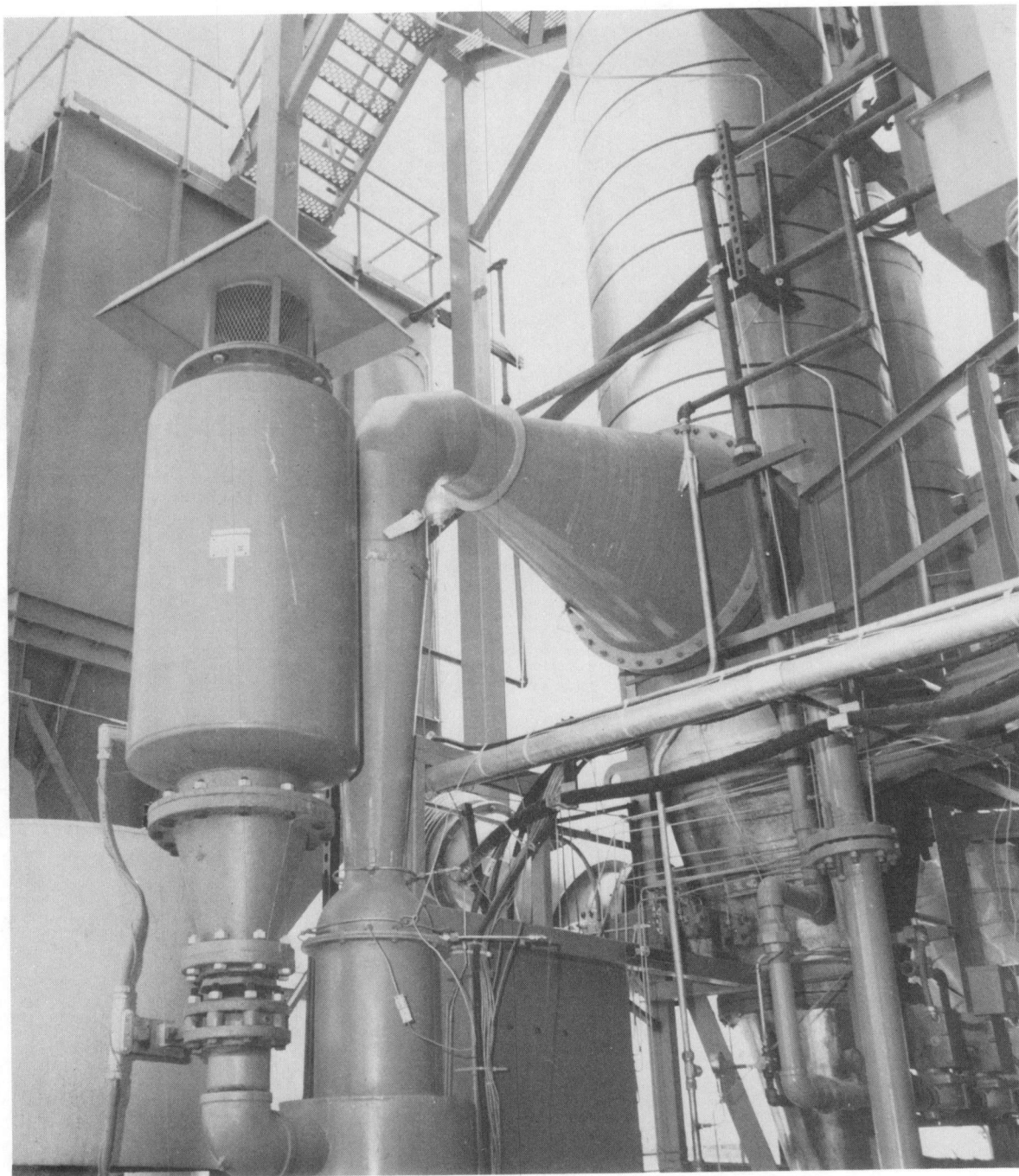
Figure C-45. Combustion Air Venturi (shown are the blowoff valve/silencer, venturi, and air preheater inlet)
