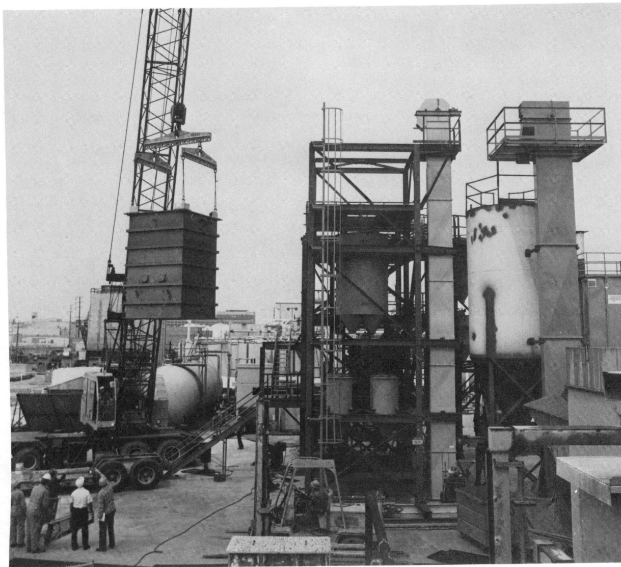
Figure C-18. Freeboard Section Being Installed
