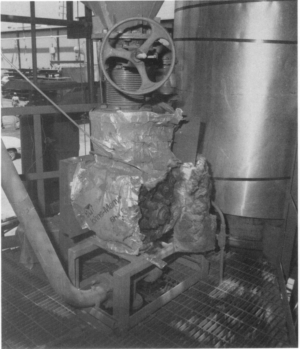
Figure C-55. Ash Recycle Rotary Valve (located under the two ash recycle hoppers; ash is conveyed from right to left, and ash injection line is shown on left)
