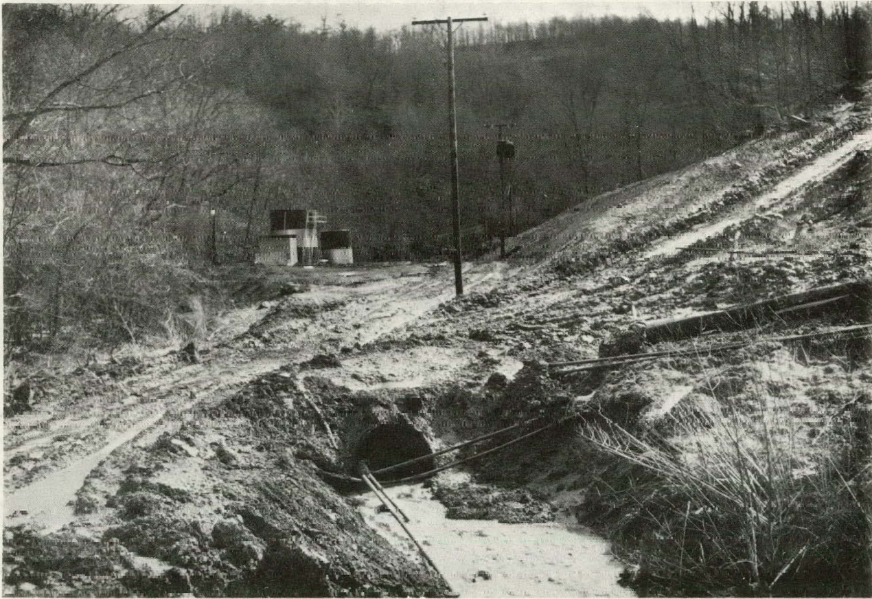
Fig. 3. Dirt access roads as a major source of erosion and stream sediment.
