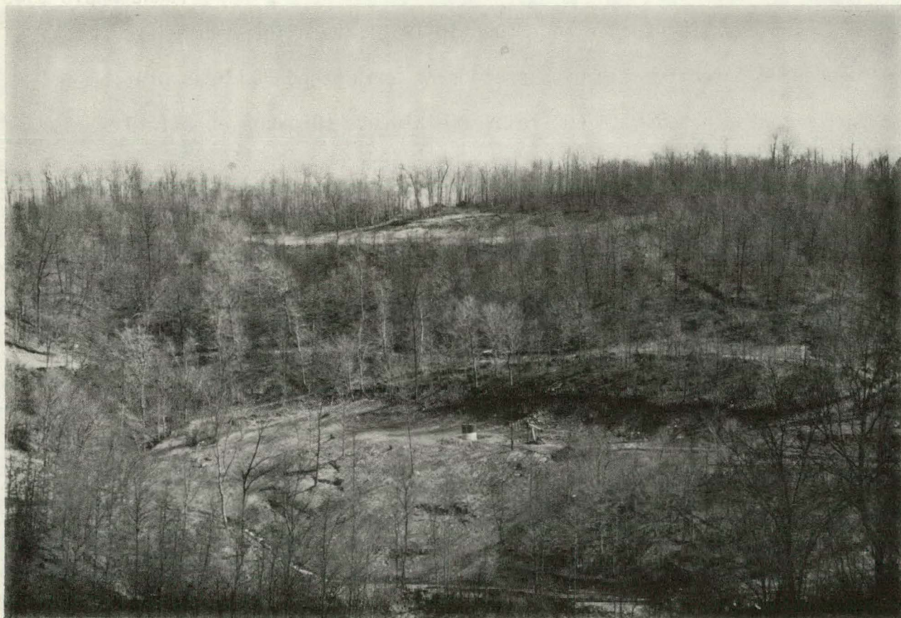
Fig. 1. Highwalls created during construction of access roads and well sites.
