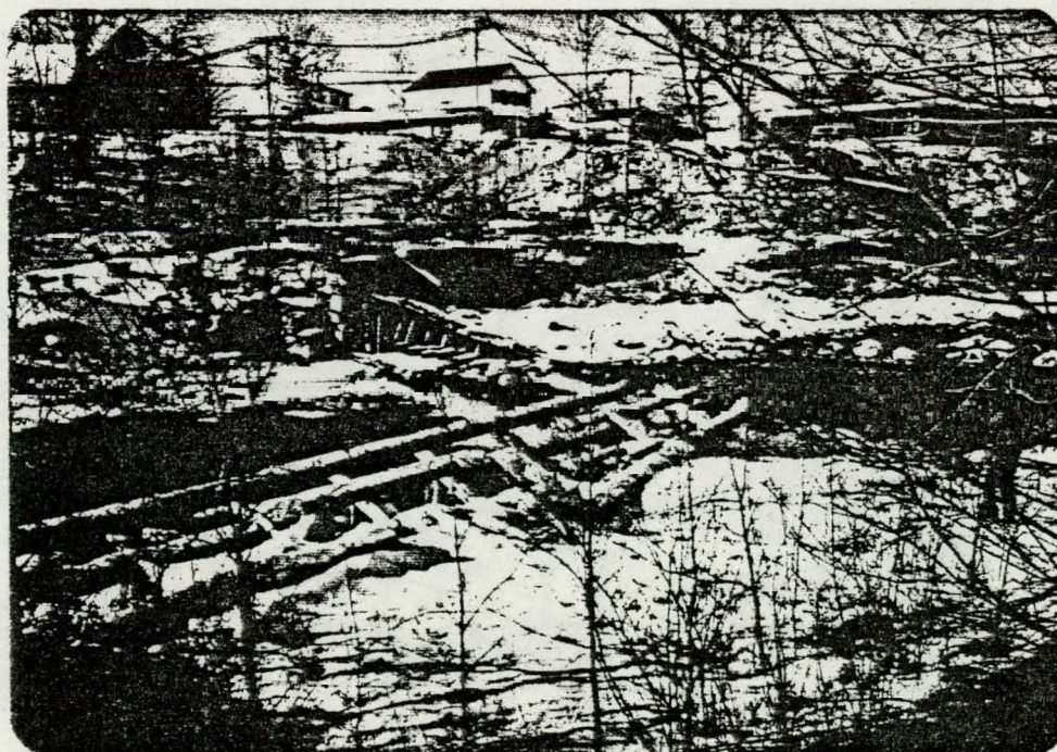
PHOTOGRAPH NO. 12 ROGERS FIBER DAM NORTH WINGWALL CRIBWORK
