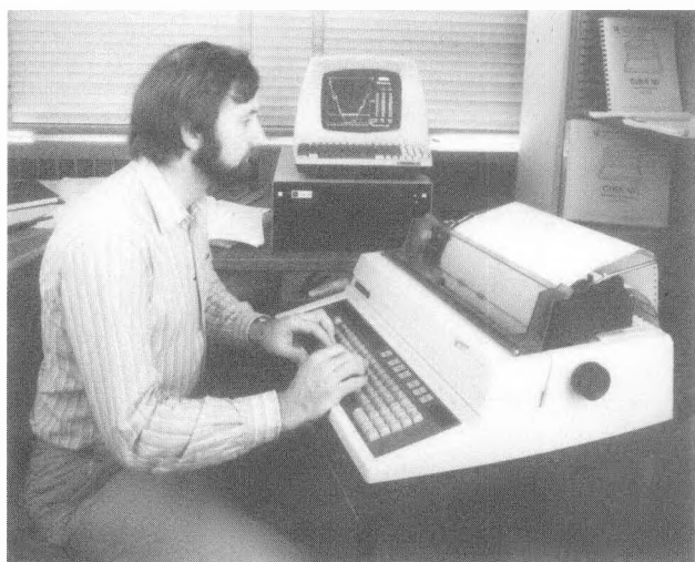
Figure 5. Viewing output from the Computerized Instrumented Residential Audit (CIRA) on a video terminal and a printer. (CBB 829-8281)
