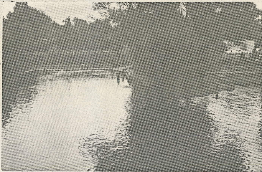
Tailwater at Union St. Dam looking upstream.
