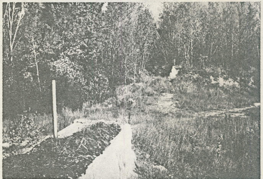
Remains of Keystone Dam looking East.
