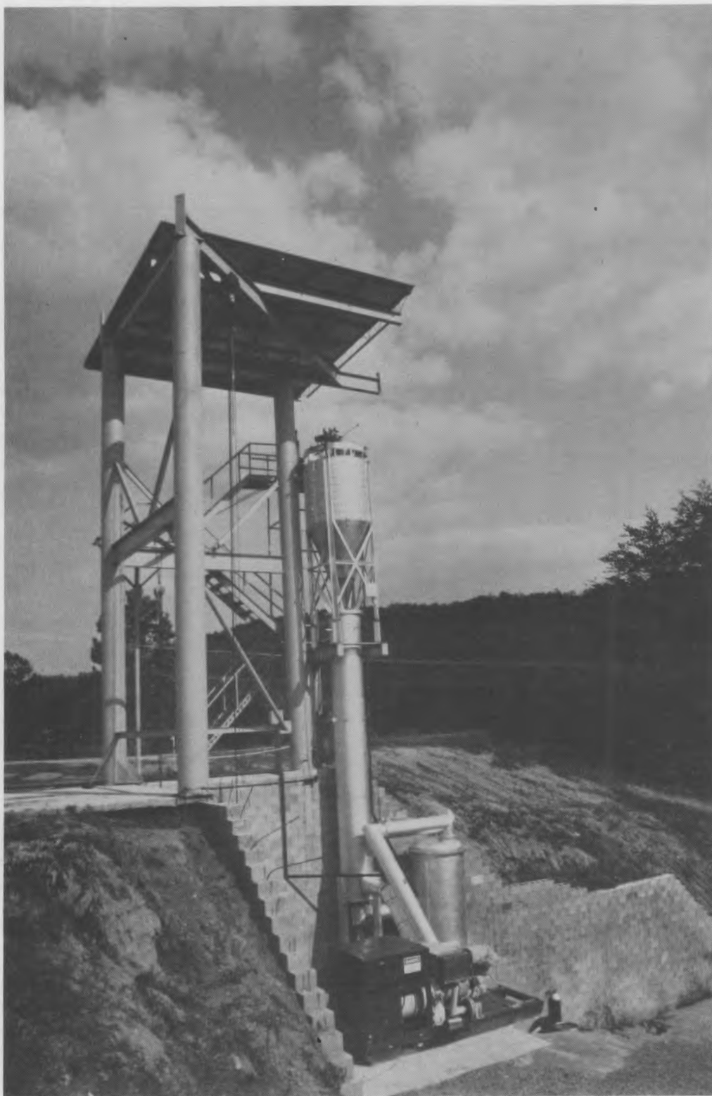
Figure 23. Wood Combustor/Gas Turbine-Generator System at Aerospace Research Corporation
