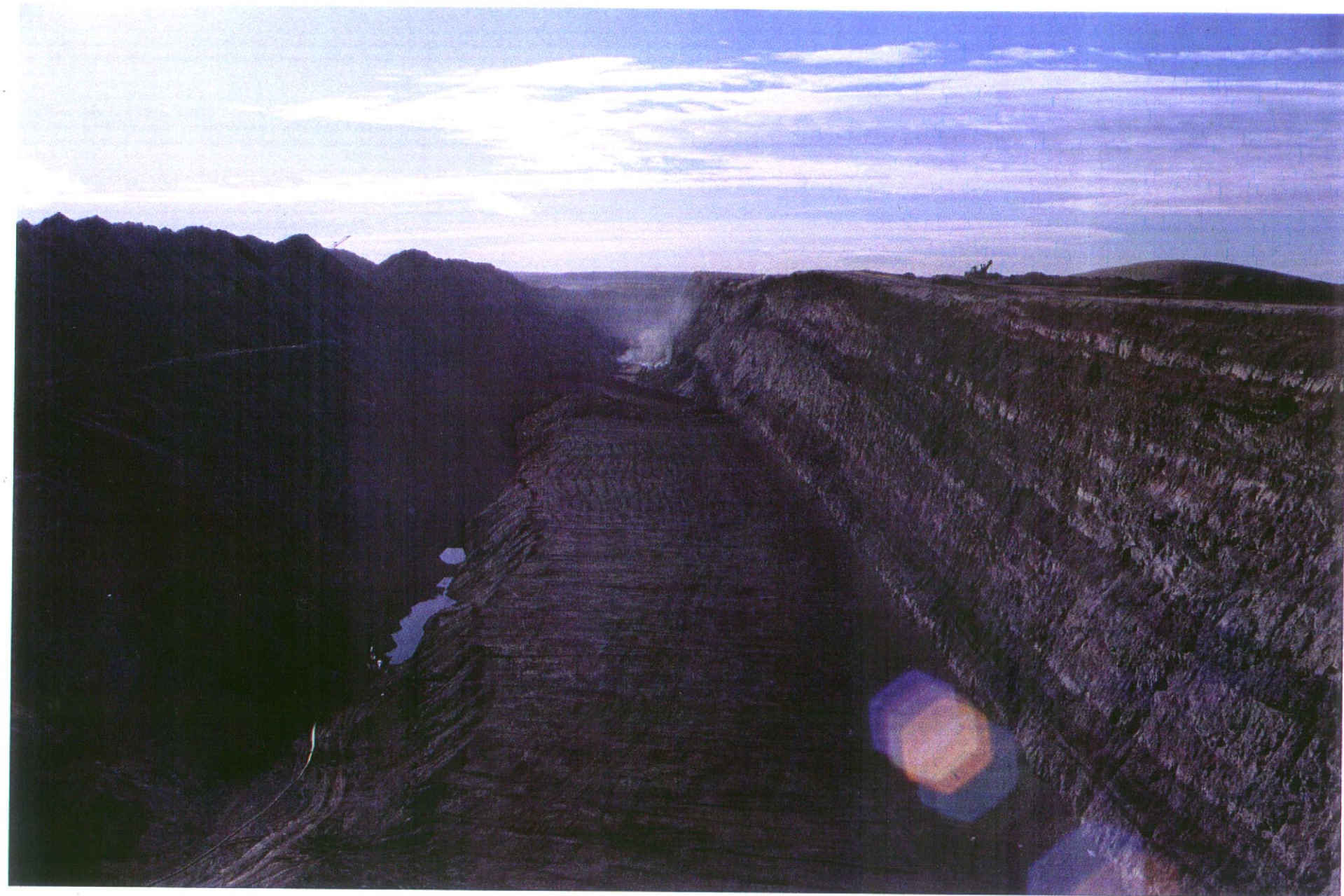
Figure 33: Black Thunder Coal Mine, WY. Overview of a pit. The overburden rock is 45-m thick, above the coal.
