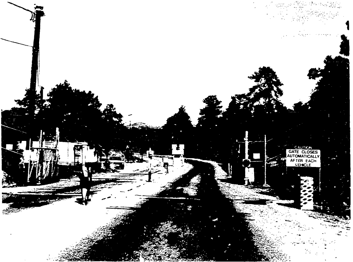
Fig. 2. LAMPF site entrance and exit gate system. The photograph shows the view when exiting the site with the gates open. Down the middle of the road are the exit badge reader, the center locking pole, the entrance badge reader, and the alarm and instrumentation shack. The radiation detector system is under the manhole cover in the center of the right exit lane.
