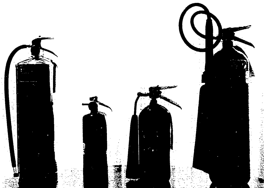
Fig. 6. Types of fire extinguishers found in MP-Division facilities. From left to right are a pressurized water extinguisher for use on paper or wood fires, a dry-chemical extinguisher for use on either Class A (paper) or Class B (flammable-liquid) fires, and CO 2 and Halon (Freon-type) extinguishers that are primarily for use on electrical fires but that also can be used on flammable-liquid fires.
