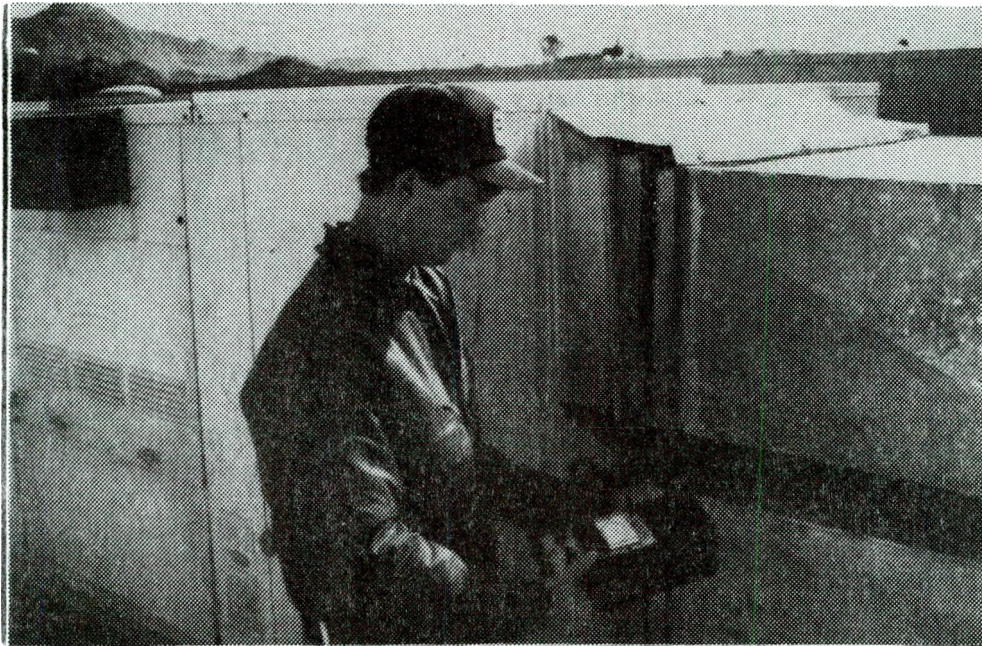
Figure 8 - Measuring Temperature of Packaged System
