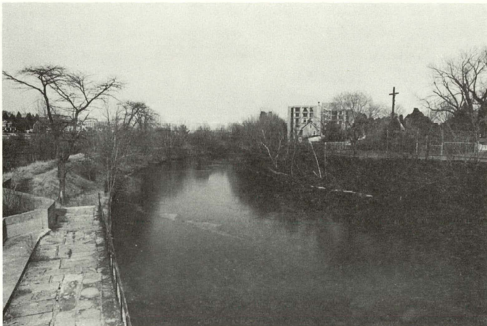
Photograph 5-2. Northern Canal Near the Gatehouse
