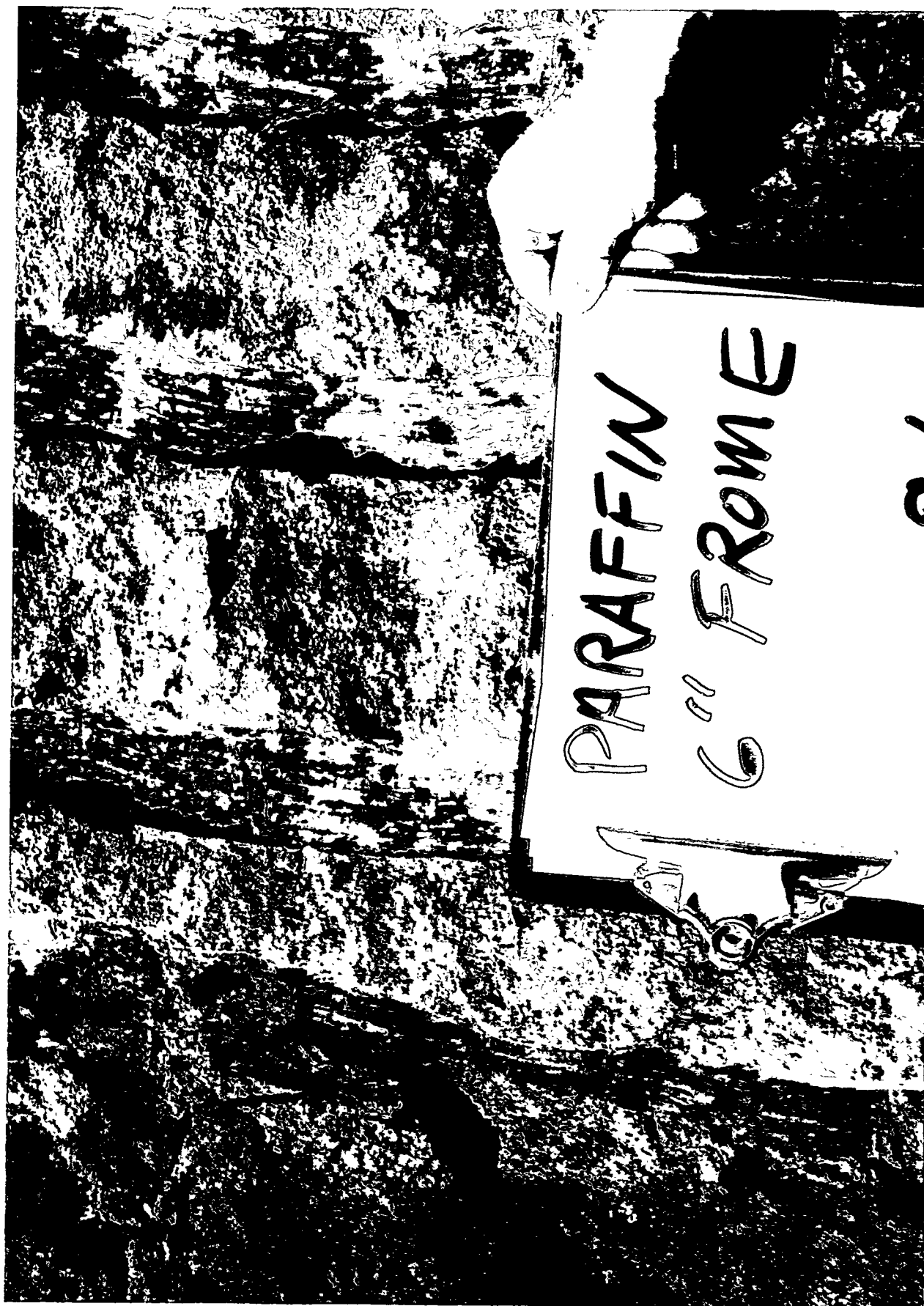
Figure 71. Paraffin pit detail at 6 in. from the east face (Photo 96-587-3-11).
