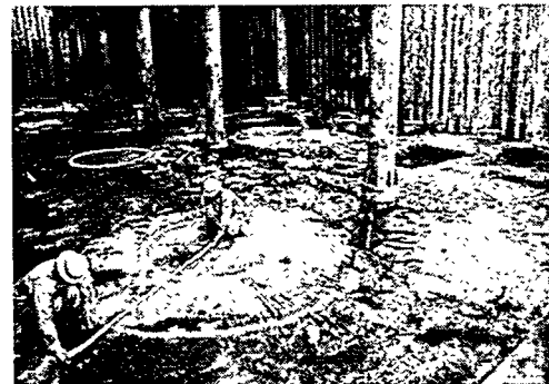
Fig.6 Underground Open Space Surrounded by Vertical Walls and Wrapping SUPERJET Piles
