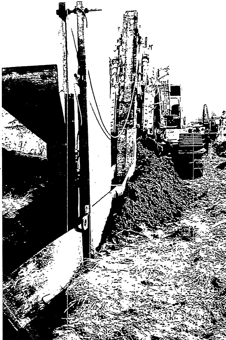
Figure 3. Shown here close-up, the HDPE panels leaving the back of the boot at the Hunter Ridge Subdivision, Jacksonville, FL.
