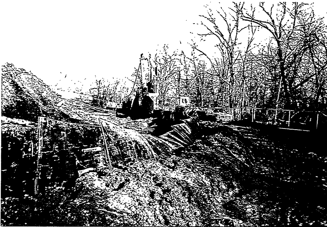
Figure 2. Waste Inc. NPL site in Michigan City, IN. GundWall panels (foreground) seen exiting the rear of the trencher (background). Collection pipe can be seen being fed in above trencher.
