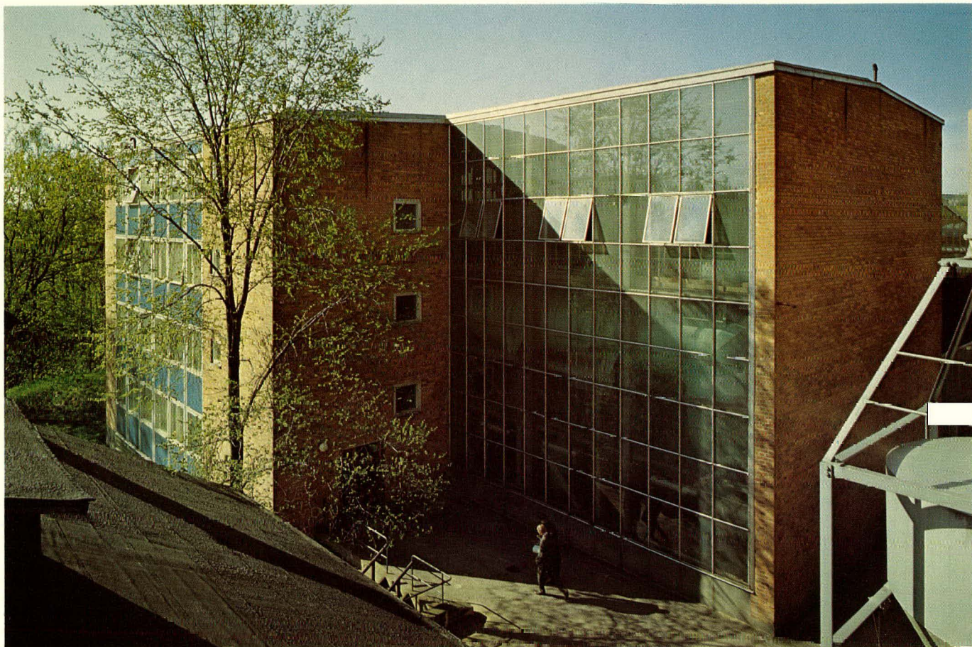
View of our modern and well-equipped turbine laboratory at Kristinehamn
