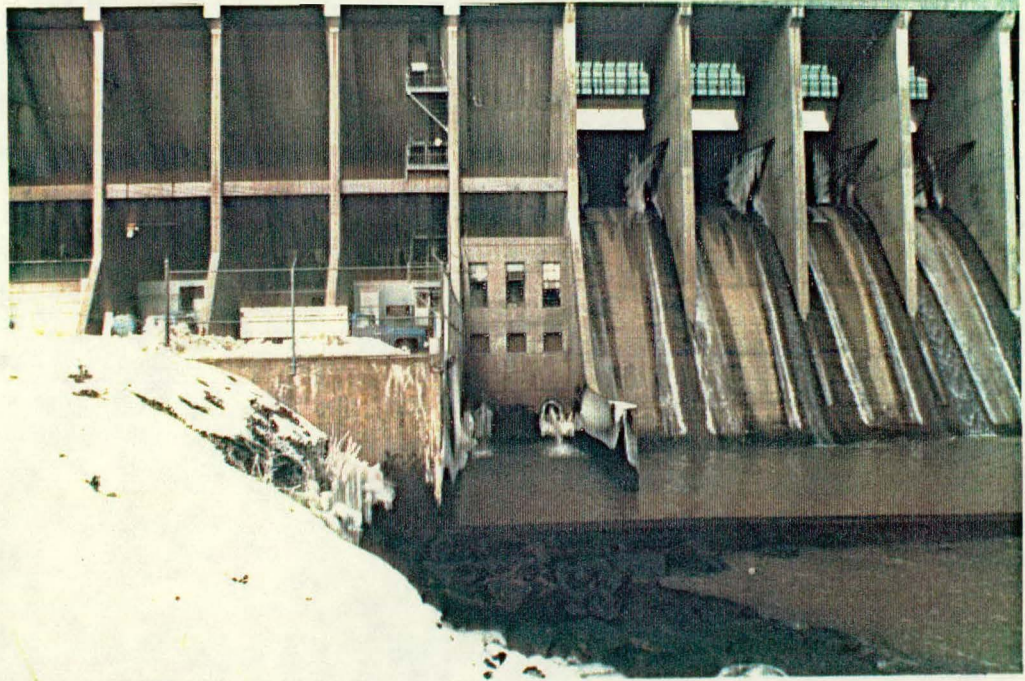
Downstream View of Powerhouse and Spillway
