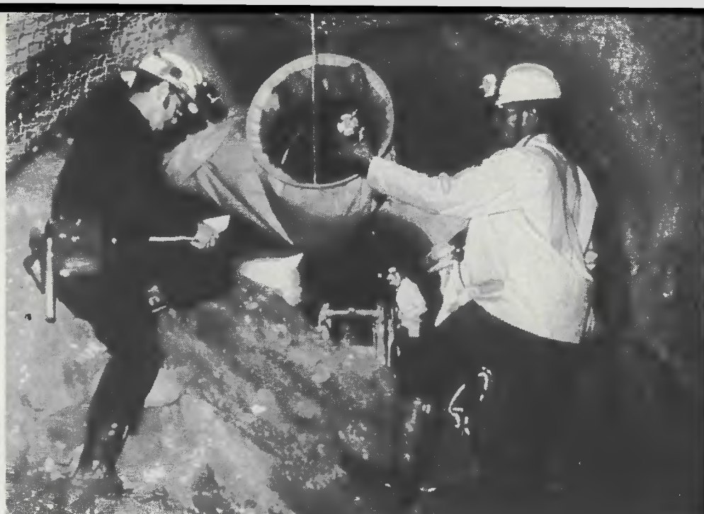
Ventilation airflow in an underground mine working area is measured by use of an anemometer.
