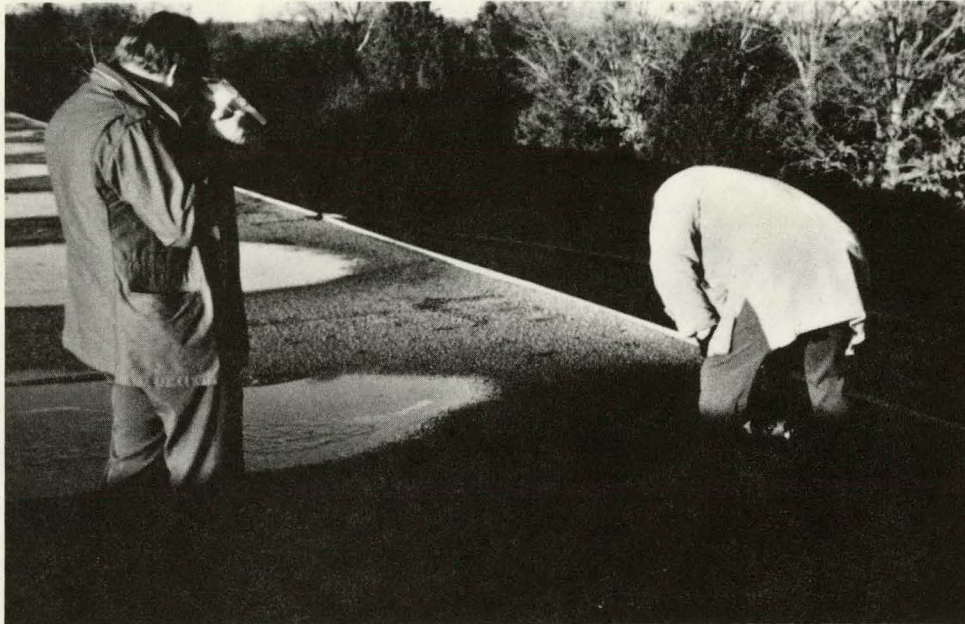
Photograph 9 shows an assistant marking areas with spray paint where the scanner has denoted heat loss through the roof.
