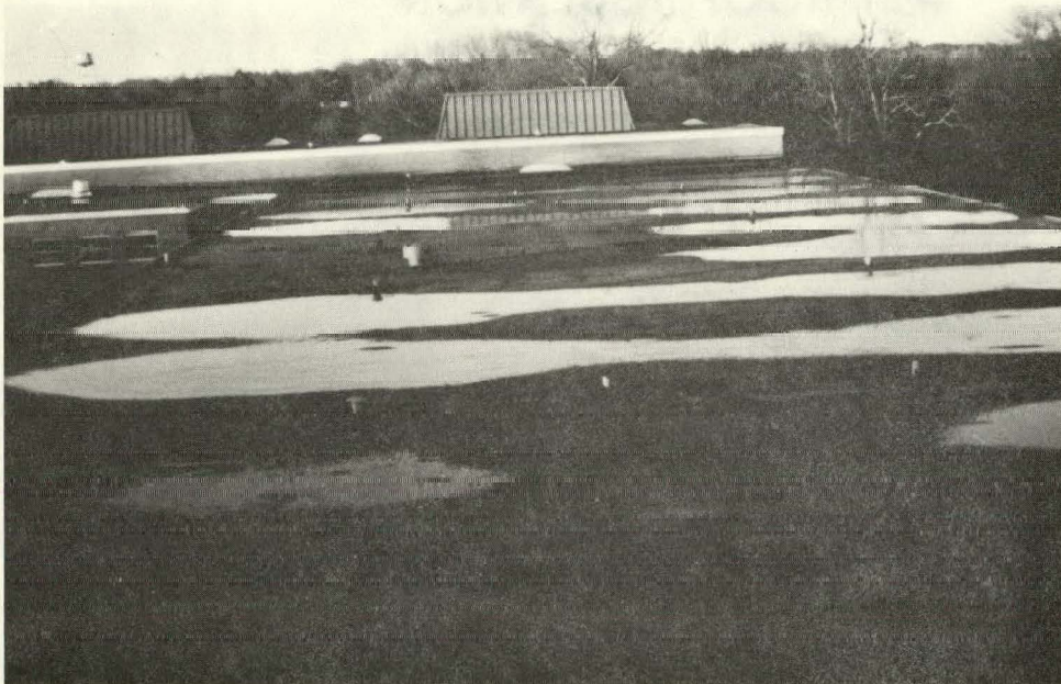
Photograph 7 shows standing water and ice on the flat roof of a school building. A roof in this condition should be checked for possible insulation damage.
