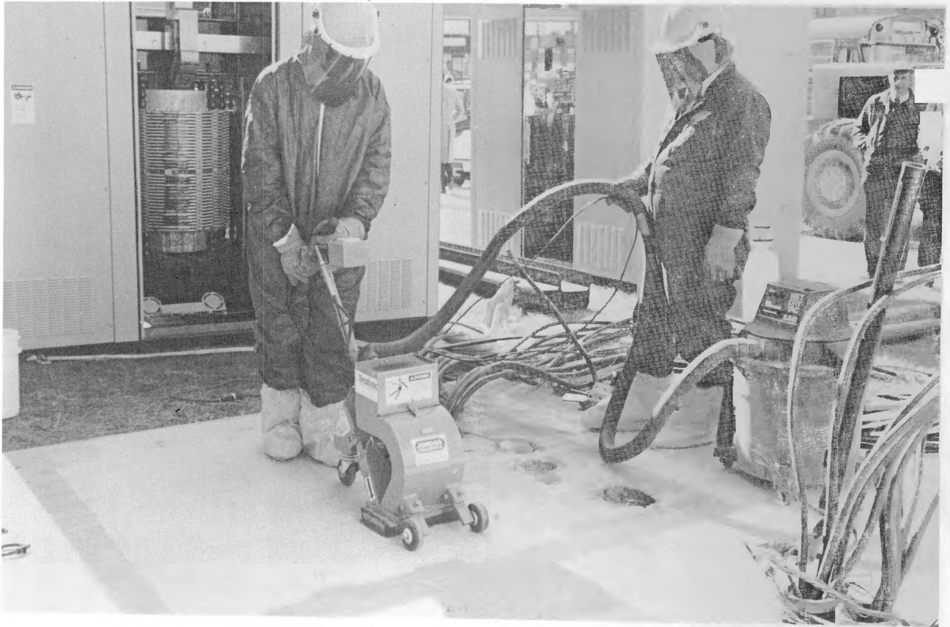
Figure 3. Concrete scarification using shotblaster.
