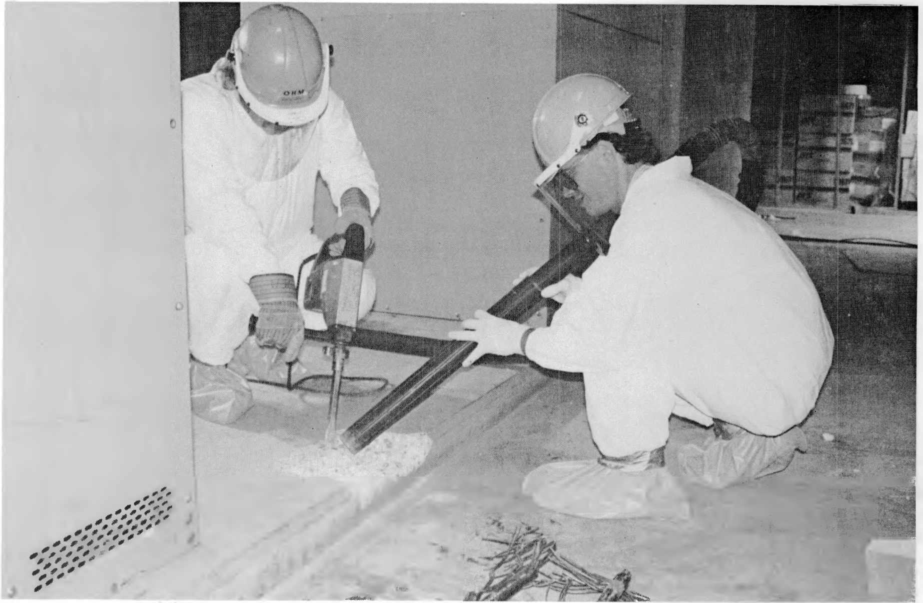
Figure 4. Concrete removal using bosch hammer.
