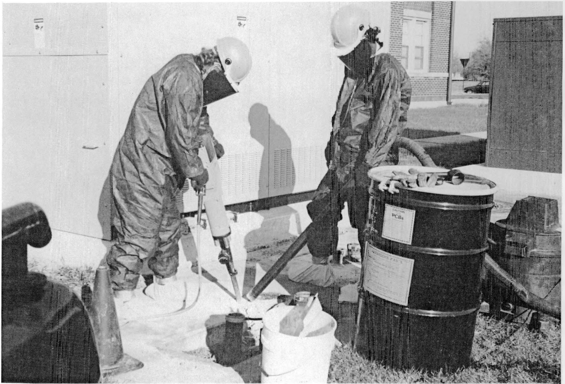
Figure 5. Concrete removal using jack hammer.
