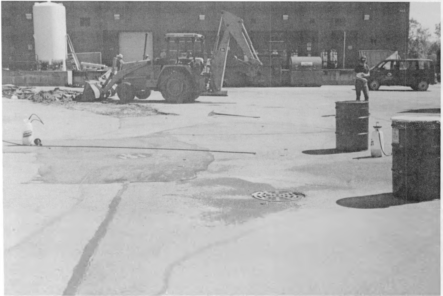
Figure 7. Pavement removal in parking area for spill cleanup.
