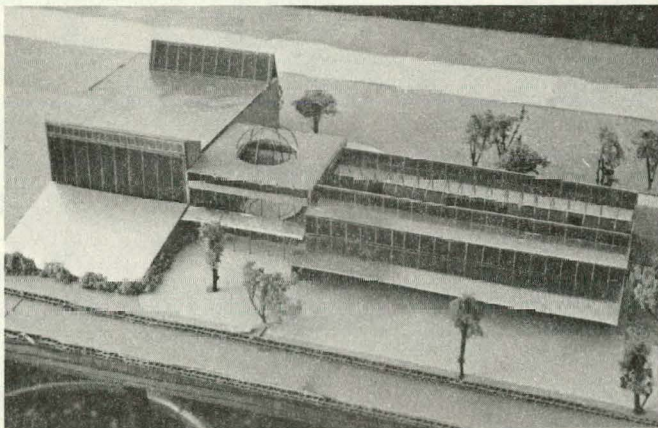
Fig. 9. Project for a cinema and office building complex. The large reflector (left) rises from grade, enhancing insolation on the vertical collector. The arriving movie-goer sees the collector mirrored in its surface. (Glare into the eyes of departing patrons is a potential problem!) Project: Mary Liang and Brent Pilip.
