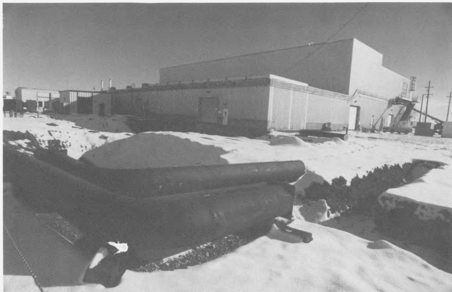
An Advanced Test Reactor Waste Heat Recovery System project at Idaho National Engineering Laboratory is having loop piping assembled as pictured, prior to being placed into the trench. Heat previously wasted in the cooling tower will be circulated through the loop to provide plant space heating.
