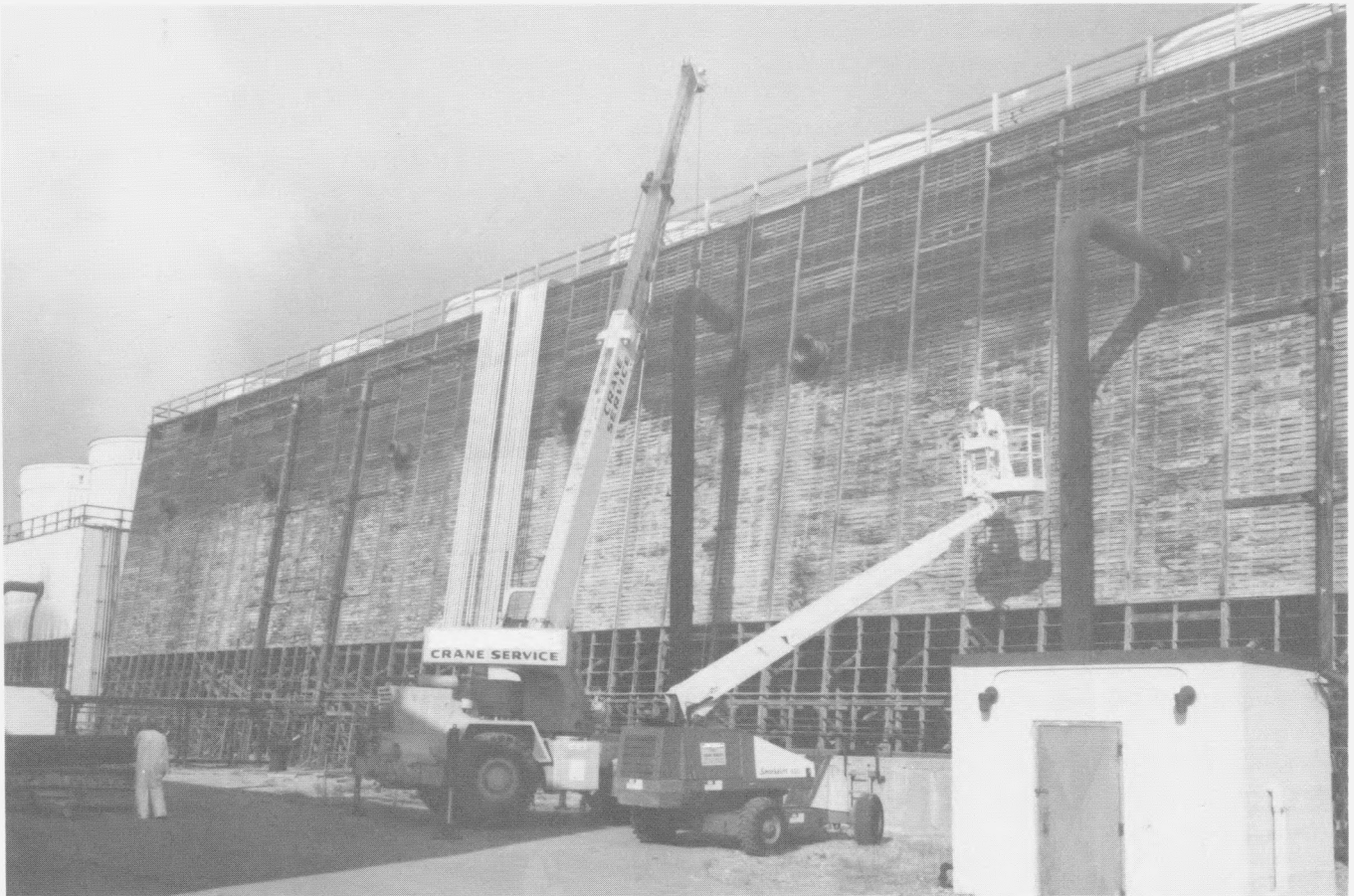
Energy efficient cooling towers replace three existing Paducah Gaseous Diffusion Plant towers. A 1000 Hp reduction will result from the completion of construction awarded in 1988.
