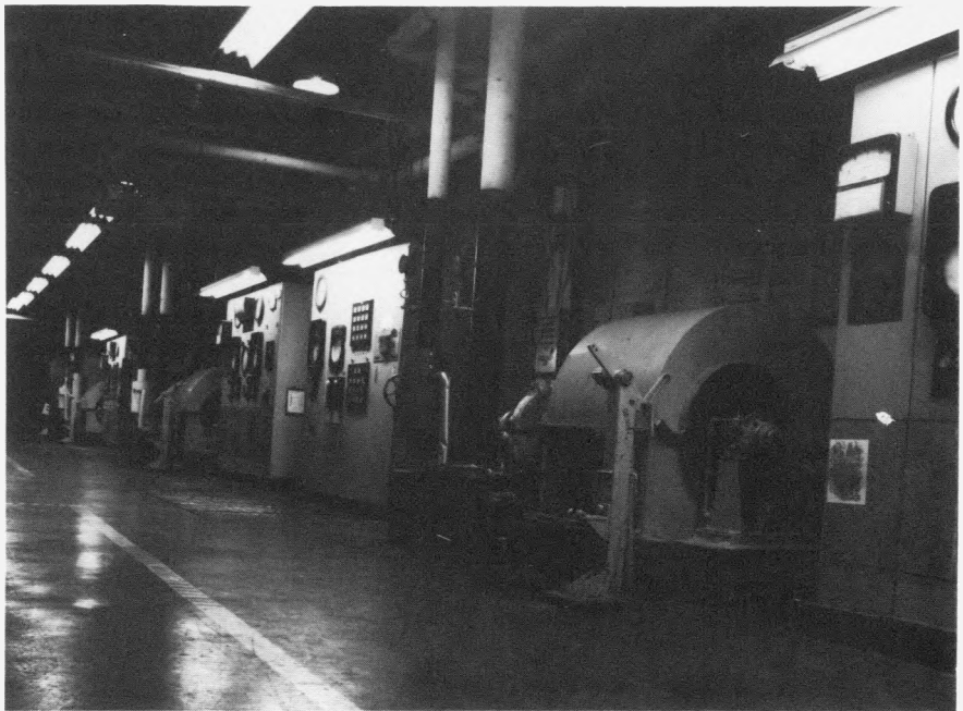
Pictured are steam plant boiler forced draft fans at the 200 E Hanford, WA Site. An In-house Energy Management funded project will install fan enclosures and ductwork for return warm air from the steam plant ceiling to the boiler inlets.
