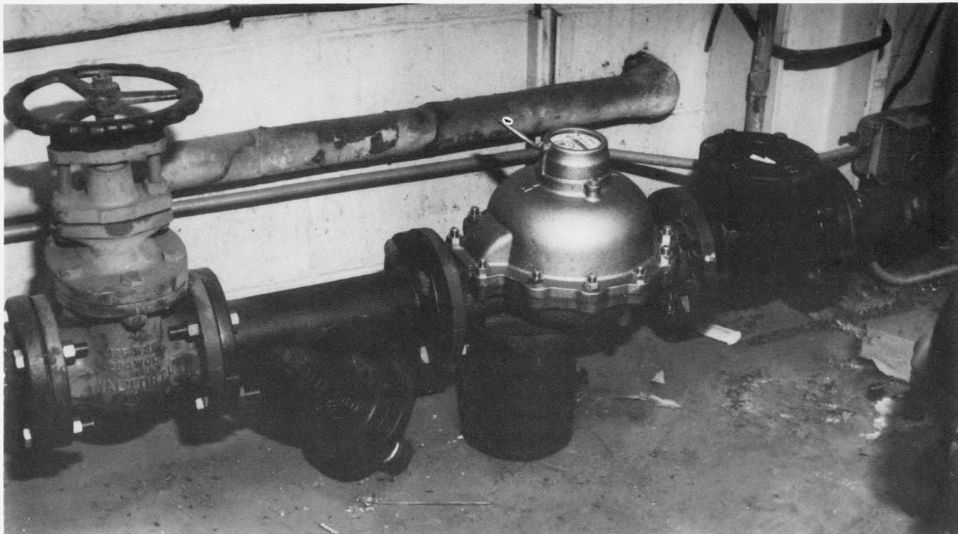
Condensate meters such as this one are being installed in buildings throughout Brookhaven National Laboratory to monitor building steam consumption.
