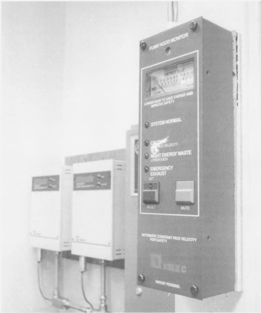
Variable speed drives like the one pictured are currently being installed on 40 laboratory fume hoods at Brookhaven National Laboratory to efficiently match exhaust fan speed to fume hood sash location.
