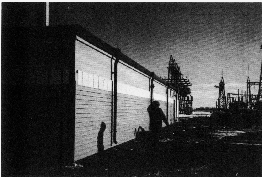
The Morris Substation in Minnesota was insulated and sided as part of the general retrofitting to make the building more energy efficient. The work is an example of some energy conservation measures Western Area Power Administration is taking.
