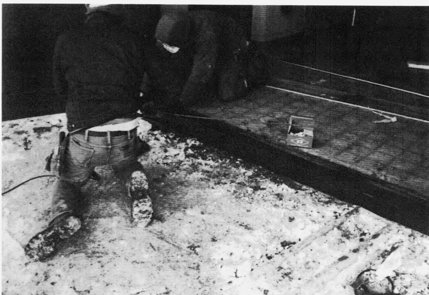
As part of the energy-efficient retrofit, 24 gauge aluminum is placed over the northwest door sill 2×6 of the Morris Substation, owned by Western Area Power Administration.
