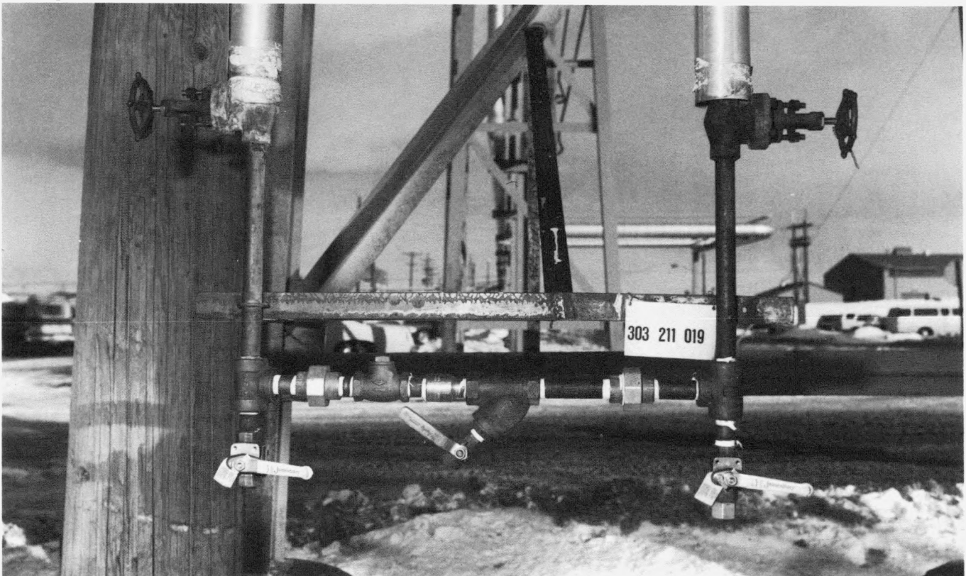
Pictured is a Steamguard Venturi nozzle steam trap installed at Rocky Flats Plant. This FY 1988 project will save about 32 billion British Thermal Units of natural gas annually when completed.
