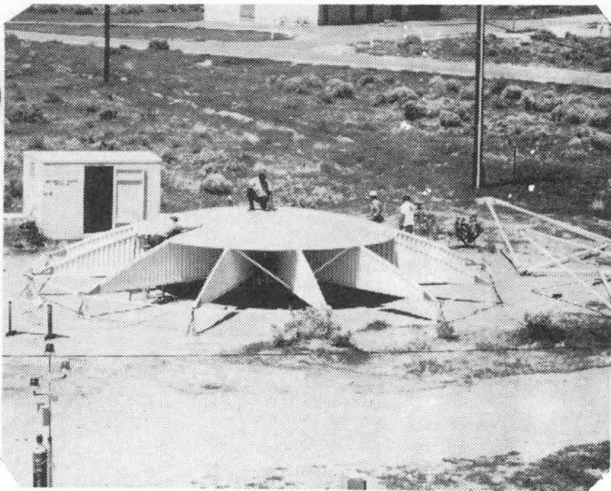
FIGURE 5. PARTIAL DISH ASSEMBLY
