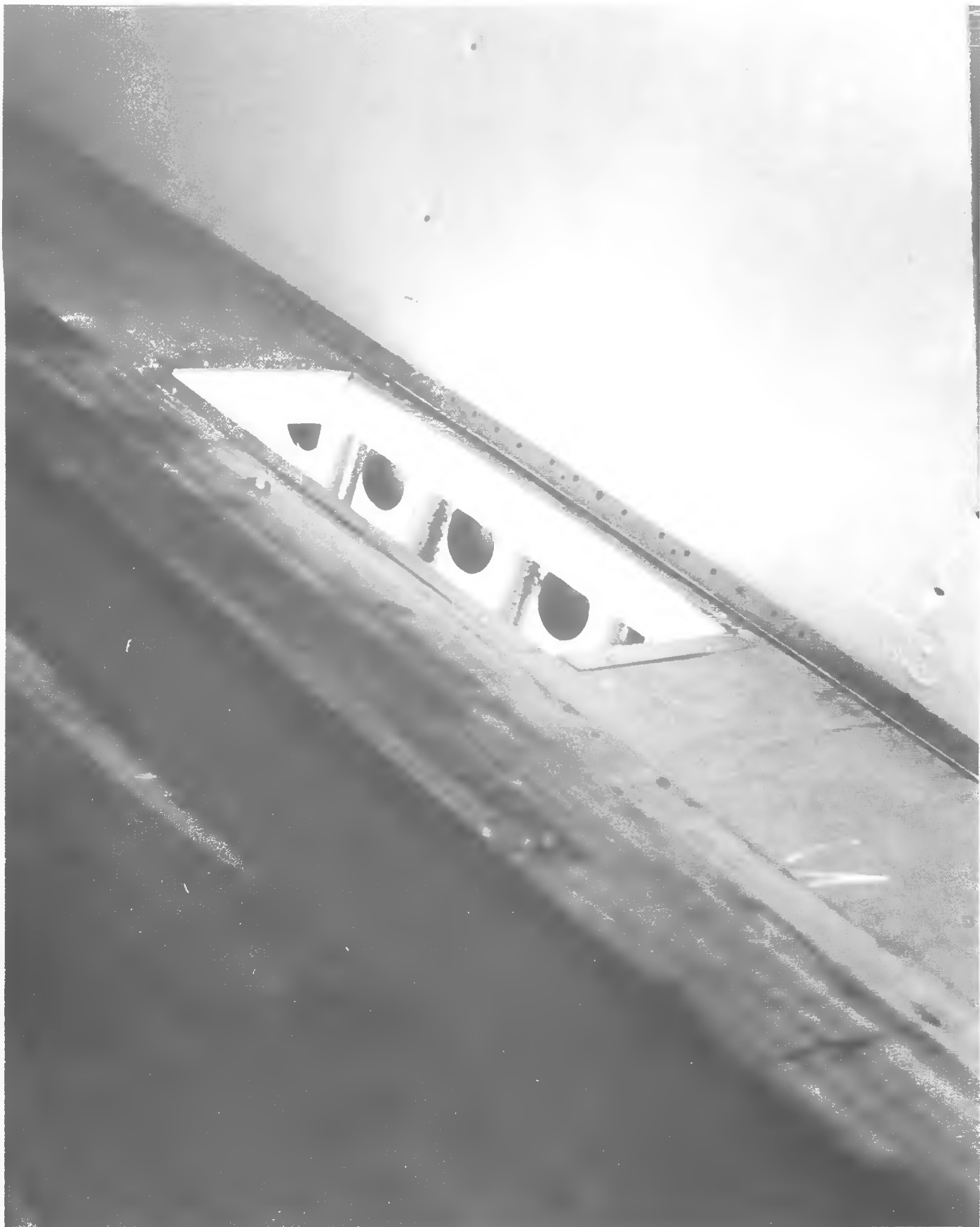
Figure 6. Air entries from plenum into radiating roof.
